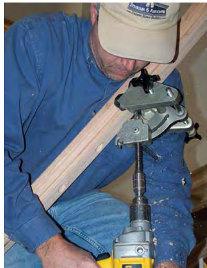
Figure 8. The author bores the balustrade holes with the help of a jig (left). A simple site-built box that fits snugly over the balusters allows him to screw each one tightly to the tread without damage (right).
