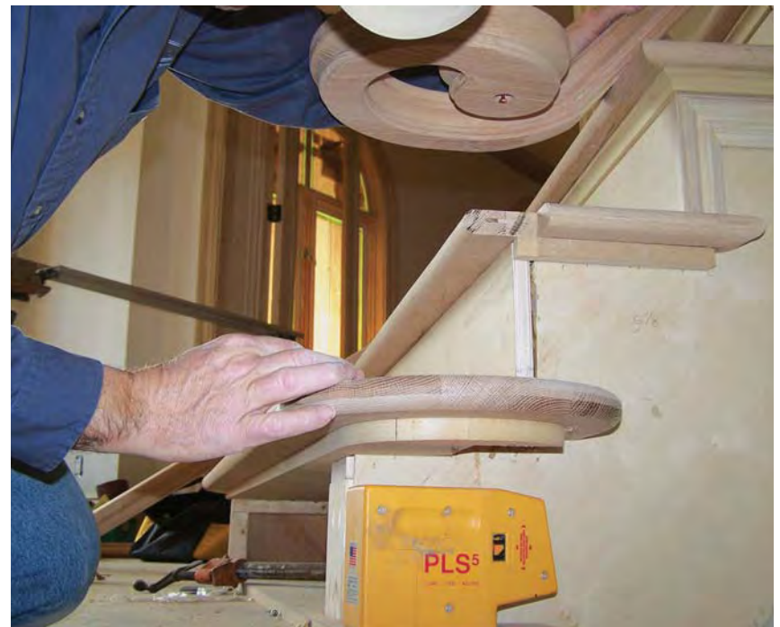
Figure 6. At the first step, a radiused subtread and matching nailer provide a form for the curved riser. Here, the author uses the laser to mark the position of the starting newel and help locate the center of the starting volute.
