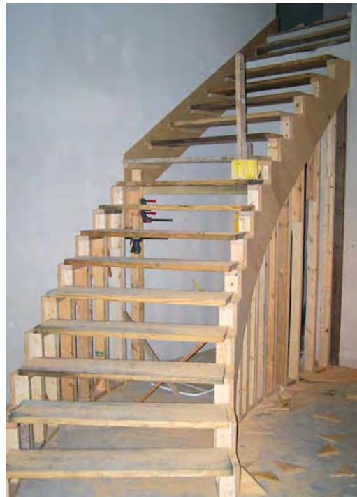
Figure 3. Along the curved layout lines, the author frames a pair of stepped walls to help support the treads (above); wall heights are taken from the story-pole layout. Each curved stringer is laminated from three layers of 5/16-inch-thick bending plywood, trimmed in place with a router equipped with a flush trim bit (far left). A final lamination of 1/4-inch birch plywood gives the stringers a smooth, paint-ready surface (left).
