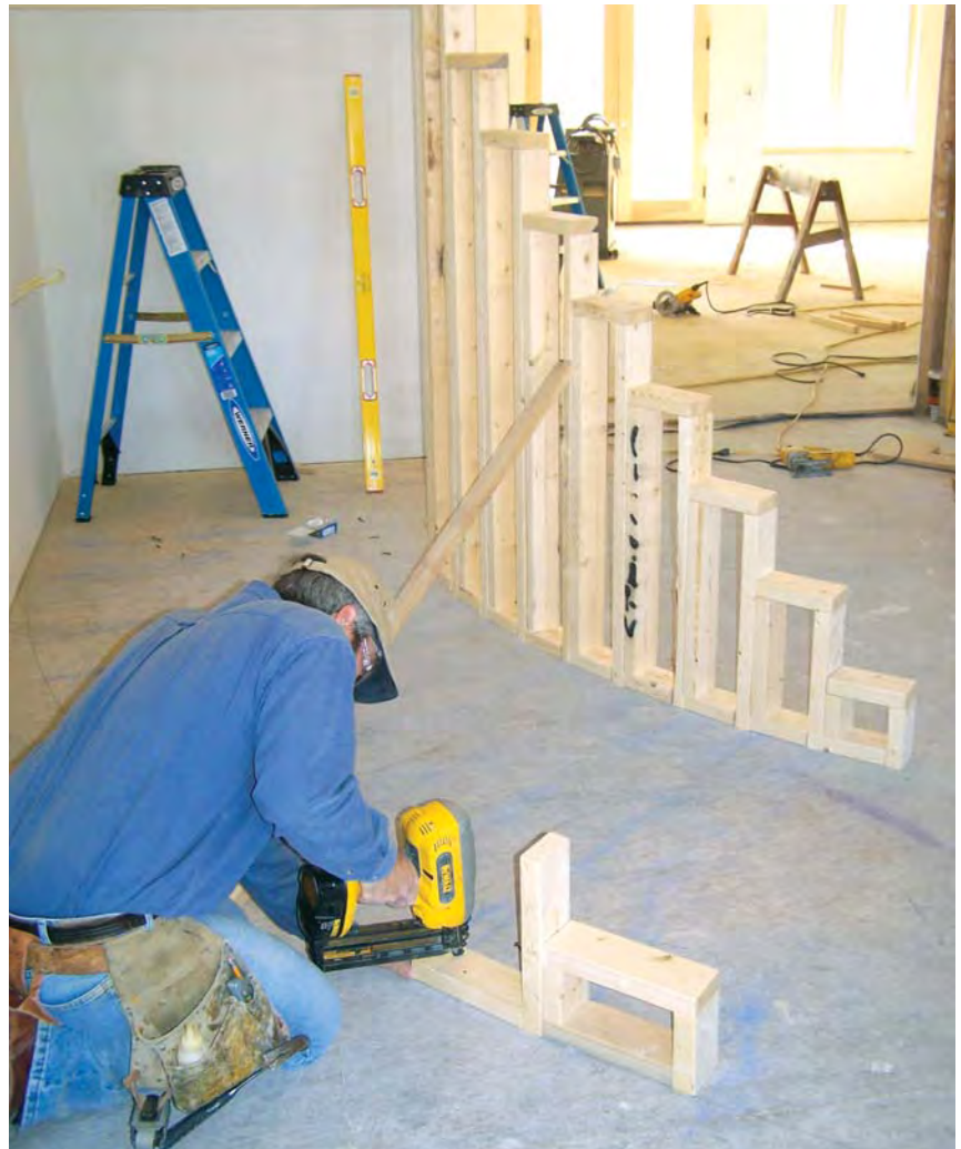
Figure 3. Along the curved layout lines, the author frames a pair of stepped walls to help support the treads (above); wall heights are taken from the story-pole layout. Each curved stringer is laminated from three layers of 5/16-inch-thick bending plywood, trimmed in place with a router equipped with a flush trim bit (far left). A final lamination of 1/4-inch birch plywood gives the stringers a smooth, paint-ready surface (left).
