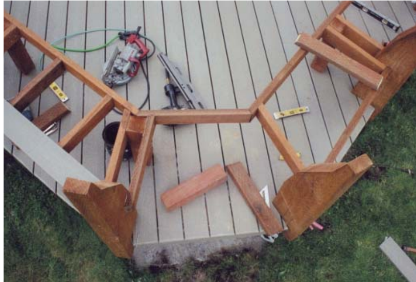
Figure 8. Allowing the 2x4s that join the front of the bench to run long made figuring the angles and lengths of the corner seat support 2x4s a matter of measurement, not complicated math.
