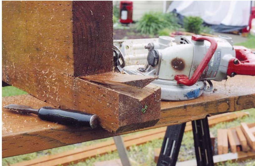
Figure 4. Two circular saws — one right-tilting and one left-tilting — are used to notch the back posts to fit the angled rim joist. A chisel cleans out the waste.
