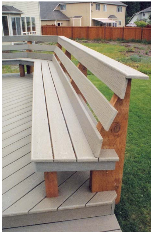
Figure 9. Installing the seat and back is the easy part, although compound angle cuts are required at the inside corners.
