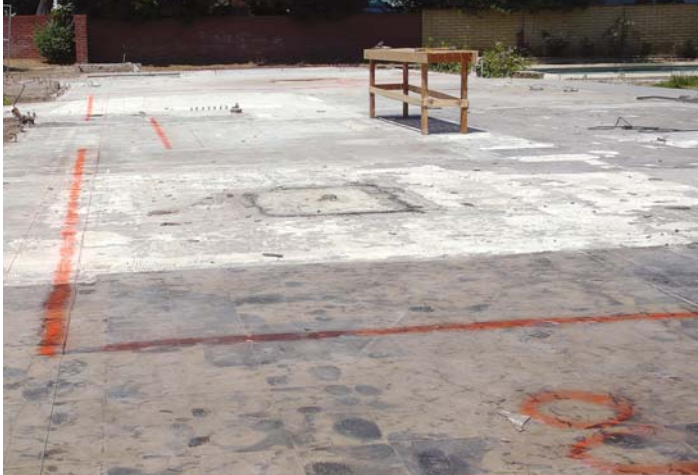
Figure 1. The placement of the new building, marked in spray paint, runs askew of the original home's layout, rendering most of the subslab footings obsolete (above). Footings and pads for the addition are laid out on the sloping lot, ready for the excavator (right).
