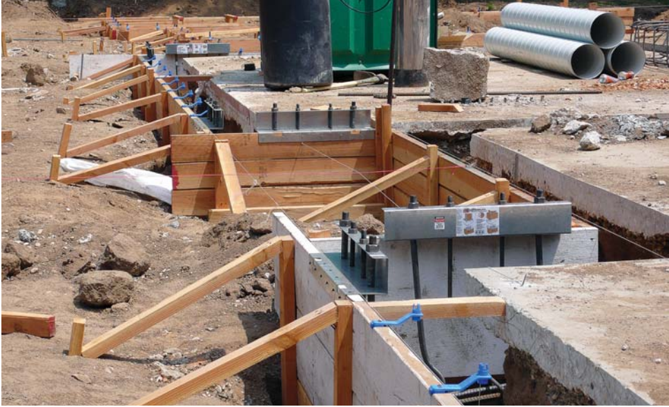
Figure 4. Formwork for the perimeter stem wall includes Simpson Strong-Wall shear-wall hold-down hardware, shown here mounted in reusable templates (left). Below, the shear panels in place.
