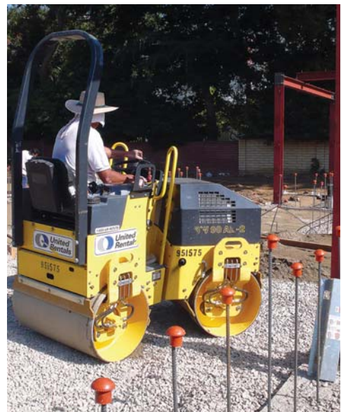
Figure 5. Though it was not required by code, the author chose to compact the gravel fill to eliminate any risk of settlement cracks forming in the slab.
