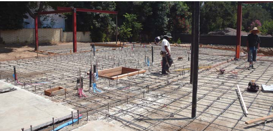
Figure 6. Rebar dowels tie new slab areas to old (left). To tie the slab to the stem walls, the crew grouted in 30-inch-long dowels on 16-inch centers. These are bent over and wire-tied to the grid (right).
