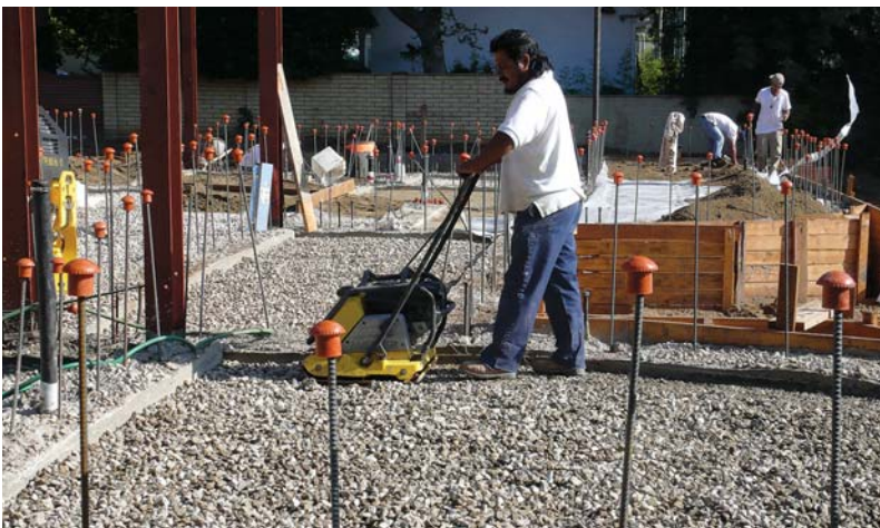
Figure 5. Though it was not required by code, the author chose to compact the gravel fill to eliminate any risk of settlement cracks forming in the slab.
