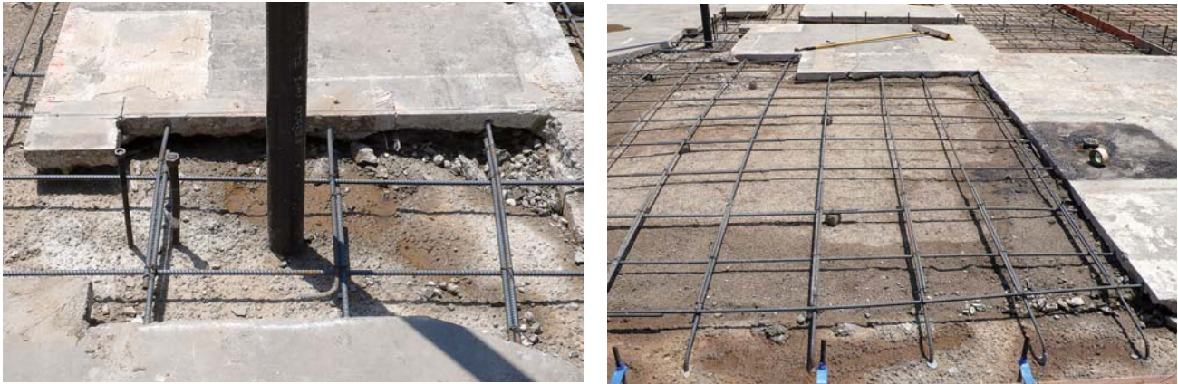
Figure 6. Rebar dowels tie new slab areas to old (left). To tie the slab to the stem walls, the crew grouted in 30-inch-long dowels on 16-inch centers. These are bent over and wire-tied to the grid (right).
