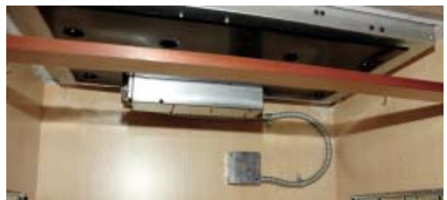
Figure 4. To allow room for the electrical connection, the drawer in this cooktop cabinet (above) stops short of the back. An electrician removes it and installs the cooktop (above right), then makes the connection with armored cable (right).
