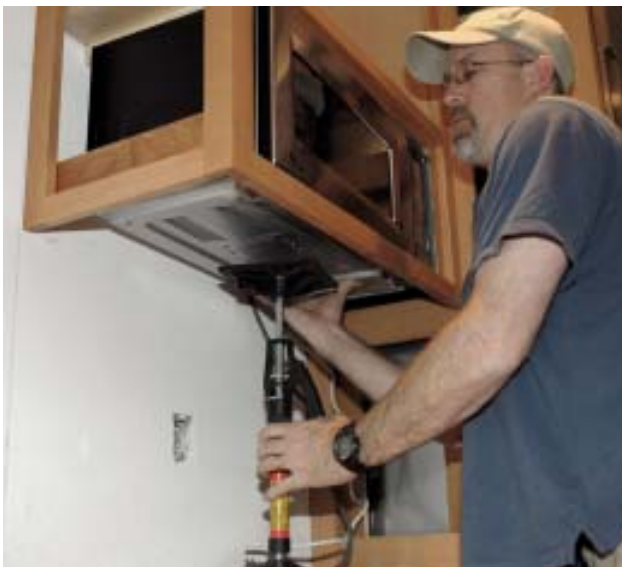
Figure 6. The author lifts a microwave into a cabinet (left), which for venting purposes will remain open from below. The microwave is held in place from above and will be plugged into a 110-volt outlet (above).
