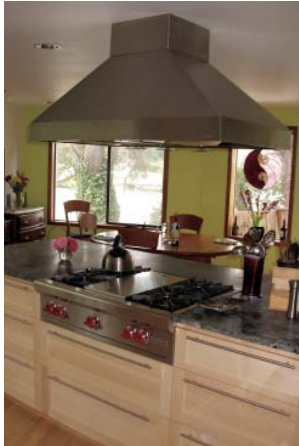
Figure 3. In the best-looking installations, a range top — which gets mounted on a custom-height cabinet — is flanked by drawers that match its height.
