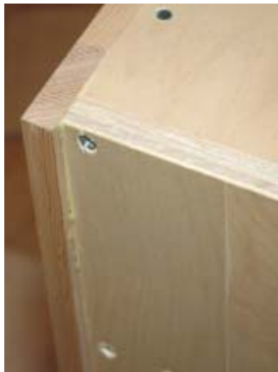
Figure 1. When installing face-frame cabinets on both sides of an appliance bay, the author measures from scribe to scribe to create the specified opening; the extra quarter inch leaves more room for the appliance itself to fit (above). Frameless cabinets (right), with their tight reveals, are less forgiving.
