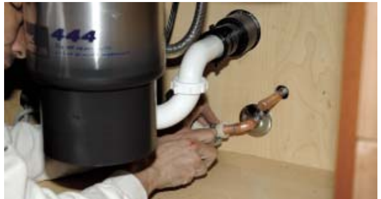
Figure 10. When customers don't want a dishwasher air-gap device on top of the sink counter, the author installs a Johnson Tee, an air-gap fitting approved by the Uniform Plumbing Code that allows a 1/2-inch copper drain line to connect directly to the ABS standpipe (left). The dishwasher drain connects to the copper drain line (below).
