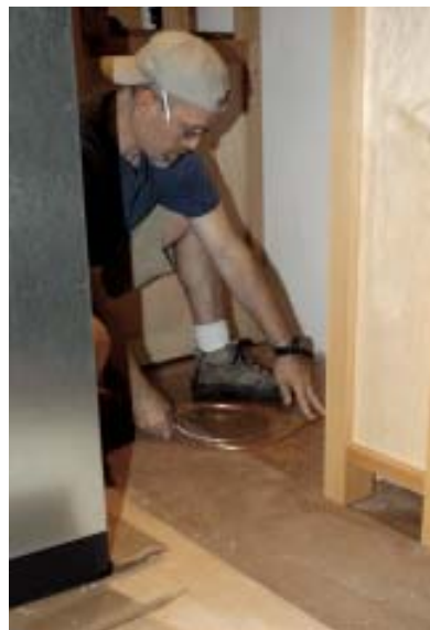
Figure 11. The author installs an anti-tip bracket for a Sub-Zero refrigerator (left). A soft copper water line (right) is run to the front of the opening, where it will connect to the icemaker.
