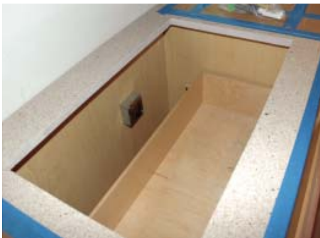
Figure 4. To allow room for the electrical connection, the drawer in this cooktop cabinet (above) stops short of the back. An electrician removes it and installs the cooktop (above right), then makes the connection with armored cable (right).
