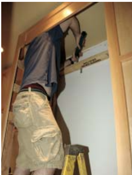
Figure 11. The author installs an anti-tip bracket for a Sub-Zero refrigerator (left). A soft copper water line (right) is run to the front of the opening, where it will connect to the icemaker.
