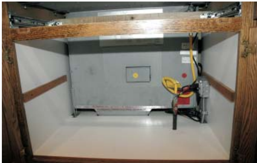
Figure 8. This downdraft vent (above) ducts through the bottom of the cabinet and connects to a remote fan and motor on the outside wall (right).
