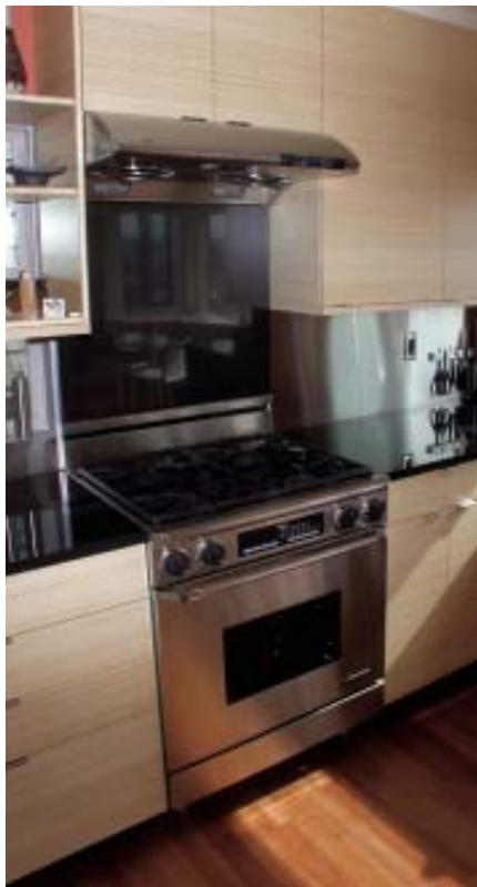
Figure 1. When installing face-frame cabinets on both sides of an appliance bay, the author measures from scribe to scribe to create the specified opening; the extra quarter inch leaves more room for the appliance itself to fit (above). Frameless cabinets (right), with their tight reveals, are less forgiving.
