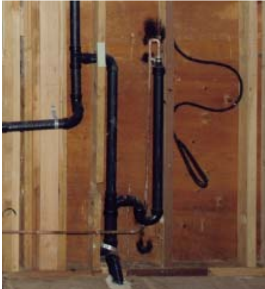
Figure 10. When customers don't want a dishwasher air-gap device on top of the sink counter, the author installs a Johnson Tee, an air-gap fitting approved by the Uniform Plumbing Code that allows a 1/2-inch copper drain line to connect directly to the ABS standpipe (left). The dishwasher drain connects to the copper drain line (below).
