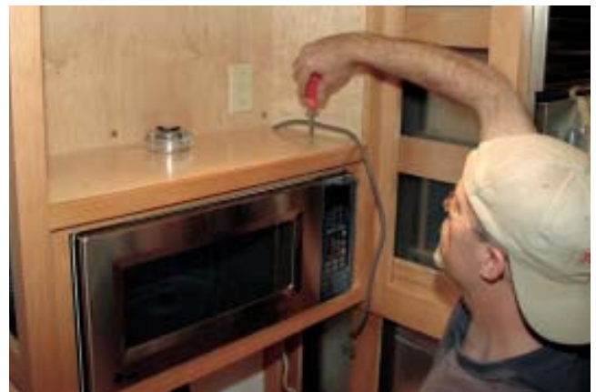
Figure 6. The author lifts a microwave into a cabinet (left), which for venting purposes will remain open from below. The microwave is held in place from above and will be plugged into a 110-volt outlet (above).
