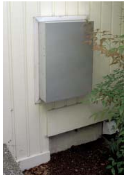
Figure 8. This downdraft vent (above) ducts through the bottom of the cabinet and connects to a remote fan and motor on the outside wall (right).
