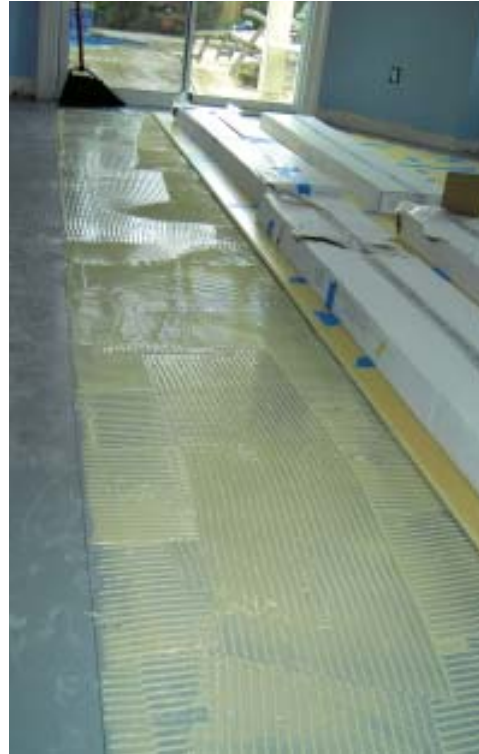
Figure 6. The slab in this room had an MVER of more than 3 pounds, so the author sealed it by troweling on a layer of Bostik's MVP4 barrier membrane (above left). This reduced vapor emission enough that he could glue down bamboo flooring with a compatible Bostik adhesive (above).
