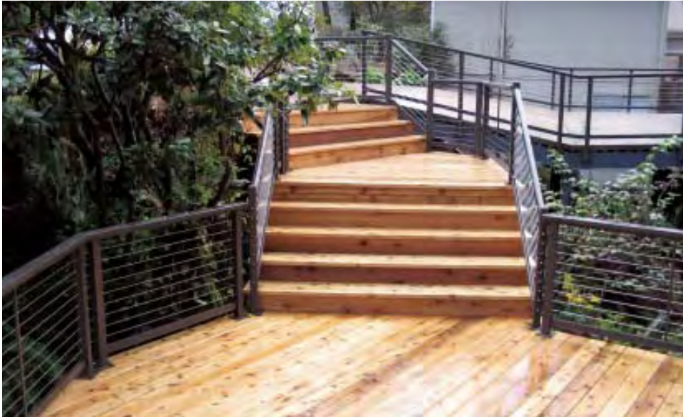
Figure 1. Although wood is the most common material for posts, powder-coated steel and aluminum are clean-looking alternatives and can be engineered to withstand the forces involved with cable railing.
