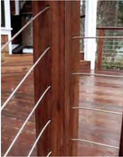
Figure 3. There are two ways to handle a single-post corner (left). One is to drill a curved hole through the post (A). Because there's a lot of tension on the inside corner of wood posts, a hardwood like ipe is recommended over soft cedar or pine for curved-hole corners. The second method is to terminate two cables at the post (B). For the cables to exit at about the same height, one of the stud holes must be drilled at an angle so it doesn't intersect the other hole (C).
