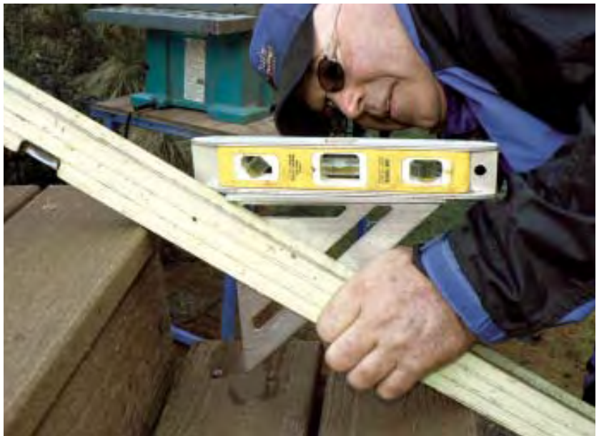
Figure 12. A long level on the tread noses establishes the stair pitch, and a Speed Square, held level, measures the stair angle (above). Use the angle to make a simple guide block for drilling cable holes in stair posts and newels (left).
