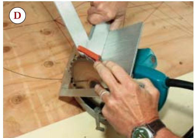
Figure 7. Pulling cut angles off the developed drawing is a matter of setting the bevel square and transferring the angles to the stock. Here, the author transfers the plumb cut for the 10/12 common (A, B) and sets the bevel angle for the 5/12 hip backing (C, D).
