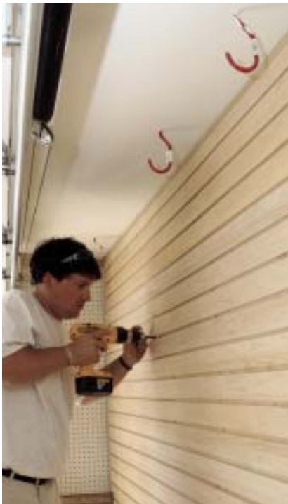
Figure 6. Installed much like lap siding, the plastic slat wall is screwed to the framing and furring with 2-inch color-matched screws. Hooks and organizing accessories are installed last.
