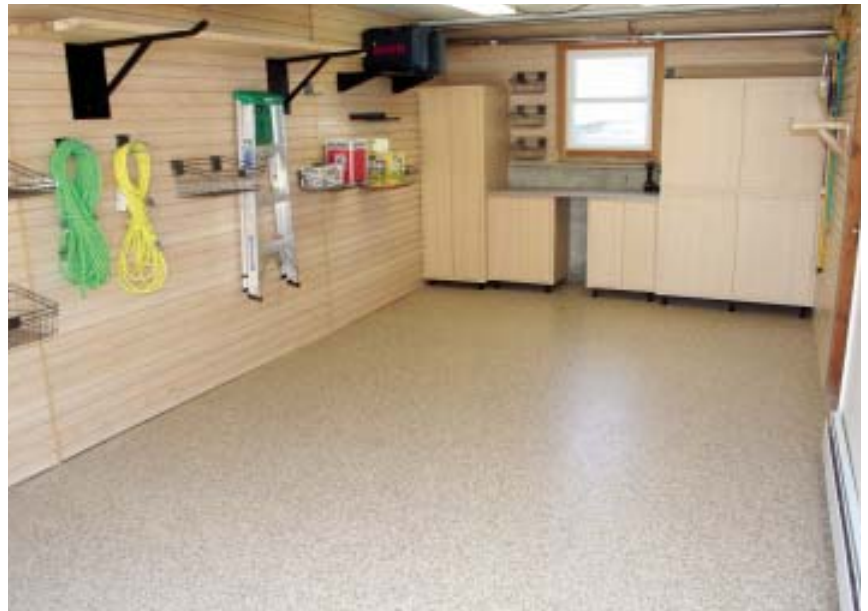
Figure 6. Installed much like lap siding, the plastic slat wall is screwed to the framing and furring with 2-inch color-matched screws. Hooks and organizing accessories are installed last.
