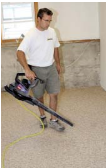
Figure 4. After excess chips are swept into a corner with a leaf blower (left), the floor is scraped in two directions to dislodge any remaining loose pieces (above).
