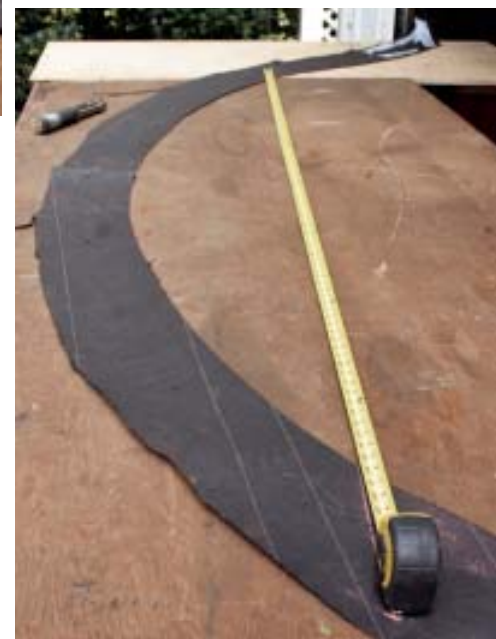
Figure 2. The author reassembles the two felt-paper sections using the plumb cut (left) and the measurement between the two reference points (below).
