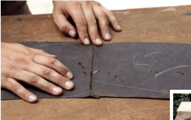
Figure 2. The author reassembles the two felt-paper sections using the plumb cut (left) and the measurement between the two reference points (below).
