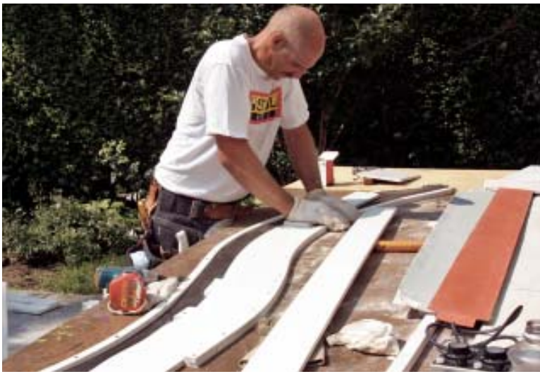
Figure 4. Once the PVC trim has been heated to 295°F, it's flexible enough to be placed in the form and molded into shape (top). The eyebrow trim is actually made up of two overlapping layers; the author forms the lower window section first (above), then the upper roof section (right).
