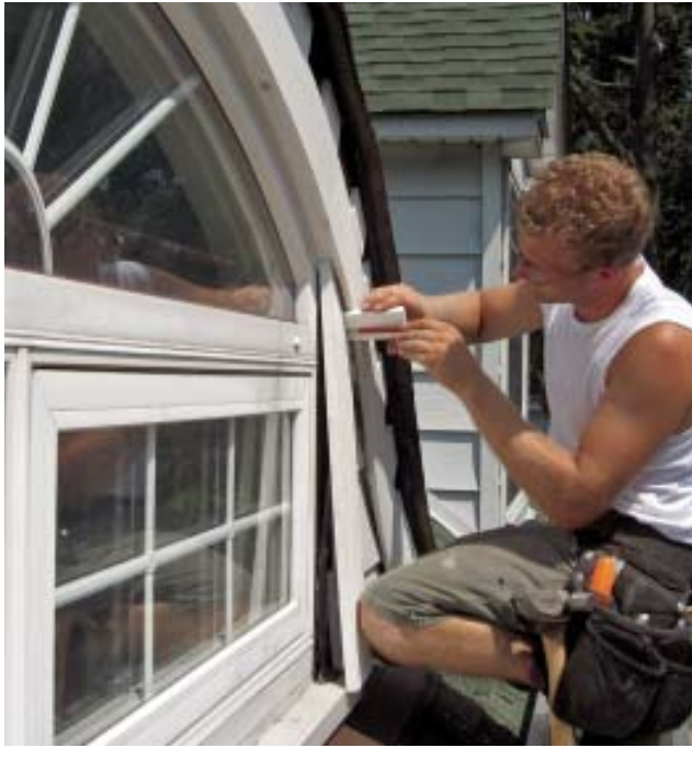
Figure 5. After fastening the lower trim layer in place with stainless-steel trim screws, a crew member scribes and fits additional PVC window trim and siding, and installs blocking to support the upper layer of trim (left). Protected by its weatherproof PVC outer layer, the eyebrow dormer is ready for another 80 years of service (below).
