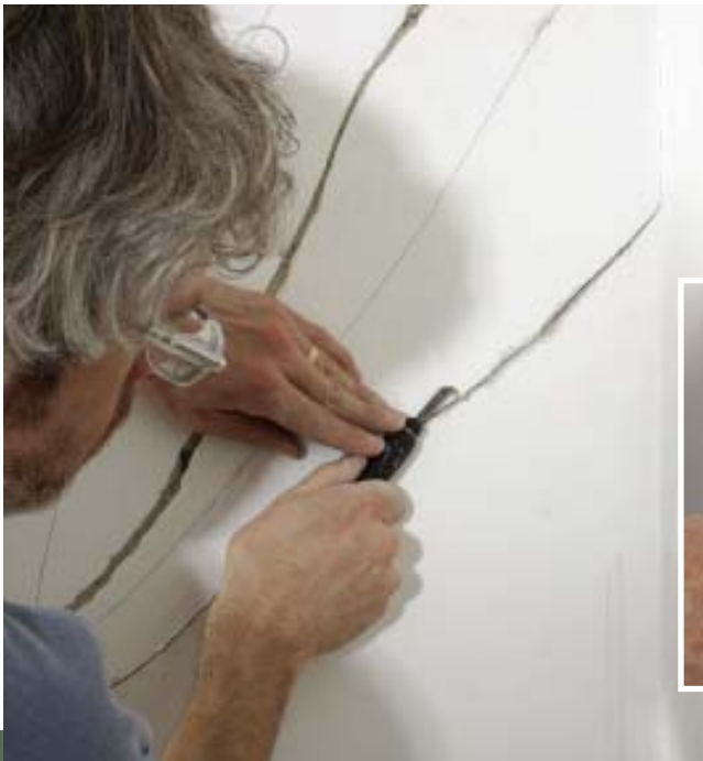
Figure 1. To fashion a strong bond between patch and plaster, it's important to widen each crack and undercut the edges to form a key. The author uses a replaceable utility knife blade to make the initial incision, breaking through the paint layers and the hard, top layer of plaster (top photos). He then employs a crack opener from Hyde Tools to enlarge the crack and undercut the edges (bottom photos).
