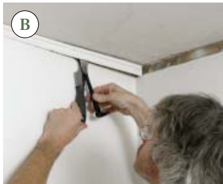
Figure 6. Ceilings that are extensively riddled with cracks are often best repaired by covering the plaster with a new layer of drywall. In preparation, the author removes existing crown by scoring the paint line with a utility knife (A) and carefully prying up the molding (B) so it can be reinstalled. He takes the time to mark the ceiling joists (C), then fastens the new board with 2-inch drywall screws (D).
