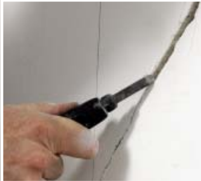
Figure 1. To fashion a strong bond between patch and plaster, it's important to widen each crack and undercut the edges to form a key. The author uses a replaceable utility knife blade to make the initial incision, breaking through the paint layers and the hard, top layer of plaster (top photos). He then employs a crack opener from Hyde Tools to enlarge the crack and undercut the edges (bottom photos).
