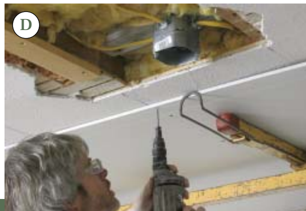
Figure 6. Ceilings that are extensively riddled with cracks are often best repaired by covering the plaster with a new layer of drywall. In preparation, the author removes existing crown by scoring the paint line with a utility knife (A) and carefully prying up the molding (B) so it can be reinstalled. He takes the time to mark the ceiling joists (C), then fastens the new board with 2-inch drywall screws (D).
