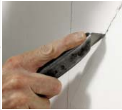
Figure 1. To fashion a strong bond between patch and plaster, it's important to widen each crack and undercut the edges to form a key. The author uses a replaceable utility knife blade to make the initial incision, breaking through the paint layers and the hard, top layer of plaster (top photos). He then employs a crack opener from Hyde Tools to enlarge the crack and undercut the edges (bottom photos).
