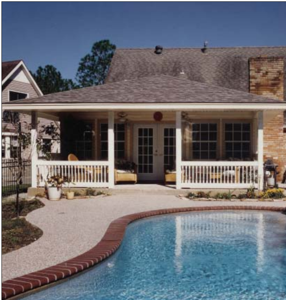
In Friendswood, Texas, GB General Contractors added this 20- by 20-foot exercise room with a covered porch that provides a shaded view of the pool.
