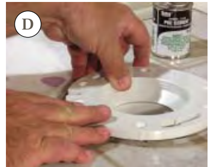
Figure 5. This plastic replacement flange has an expandable gasket, allowing it to be used with both cast-iron and plastic pipe (A). Replacement flanges also come in various diameters to fit 3- and 4-inch PVC and ABS drainpipe (B). After priming and applying cement to the fitting and the drain (C), the author inserts the new flange (D).
