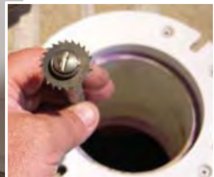
Figure 3. The author uses a small shaft-mounted saw blade powered by an electric drill (above) to separate a plastic closet flange from its drain flooring (left).
