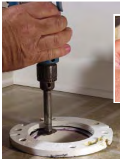
Figure 3. The author uses a small shaft-mounted saw blade powered by an electric drill (above) to separate a plastic closet flange from its drain flooring (left).
