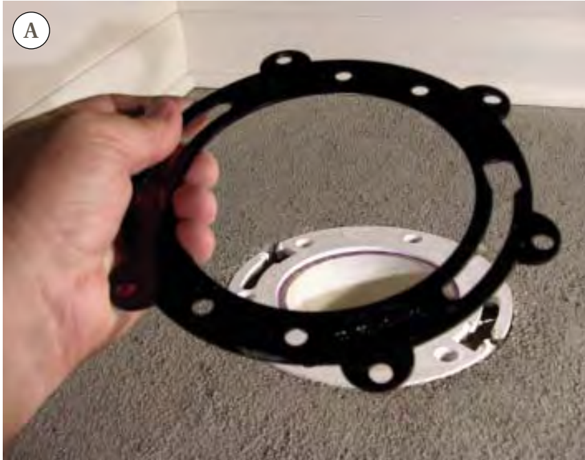
Figure 2. When both bolt slots are broken, the author installs a closet ring replacement over the existing closet flange (A). After marking and drilling holes in the slab for anchors, he applies a bead of silicone caulk (B), then positions the ring on top of the existing flange and sets the anchors (C). With the wax ring in place, the flange is ready for toilet installation (D).
