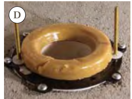
Figure 2. When both bolt slots are broken, the author installs a closet ring replacement over the existing closet flange (A). After marking and drilling holes in the slab for anchors, he applies a bead of silicone caulk (B), then positions the ring on top of the existing flange and sets the anchors (C). With the wax ring in place, the flange is ready for toilet installation (D).
