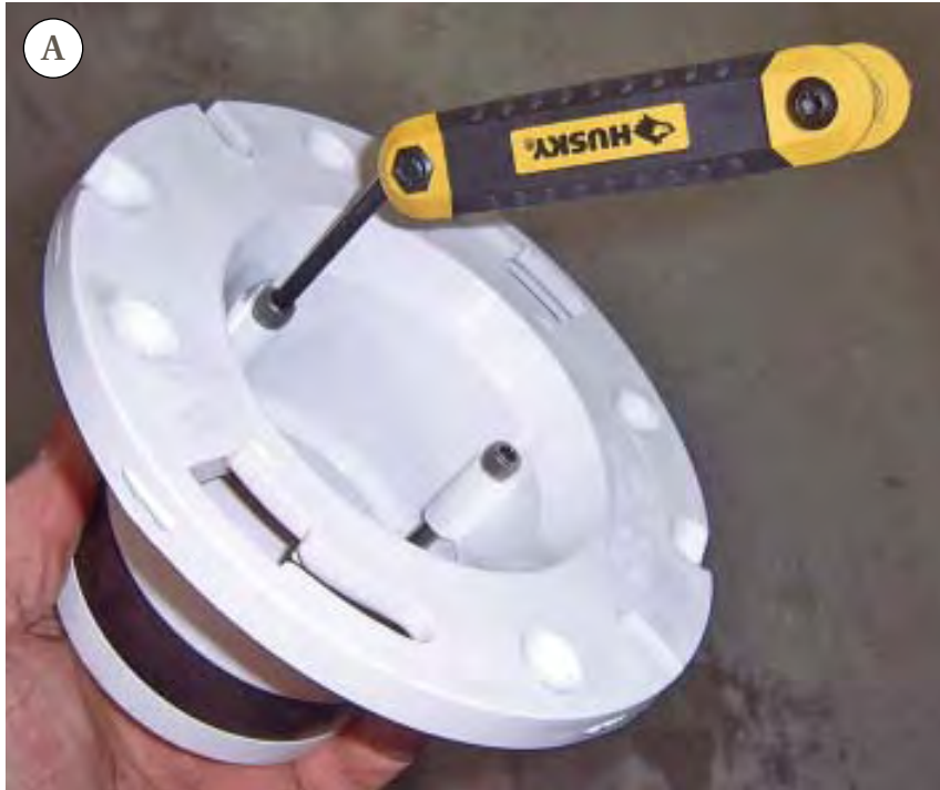
Figure 5. This plastic replacement flange has an expandable gasket, allowing it to be used with both cast-iron and plastic pipe (A). Replacement flanges also come in various diameters to fit 3- and 4-inch PVC and ABS drainpipe (B). After priming and applying cement to the fitting and the drain (C), the author inserts the new flange (D).
