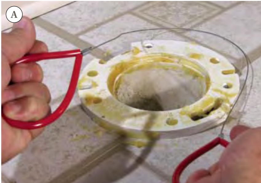
Figure 4. In cases where a closet flange is surface-mounted (rather than flush to the floor), the author slips a simple cable saw (A) under the flange and pulls it back and forth in a sawing motion to cut through the plastic (B). He removes the damaged flange (C), cleans up the cut with a utility knife (D), and then installs a replacement flange that slips inside the existing drainpipe.
