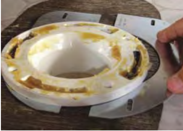
Figure 6. When there's minor damage to the flooring around a closet flange, the author reinforces the connection between the flooring and closet flange with galvanized steel flange support plates (above). He screws the plates to sound flooring either in front of or behind the flange (right) and then fastens the flange to them.
