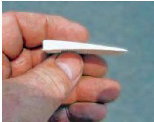
Figure 8. Plastic shims help prevent a toilet from rocking on uneven flooring.
