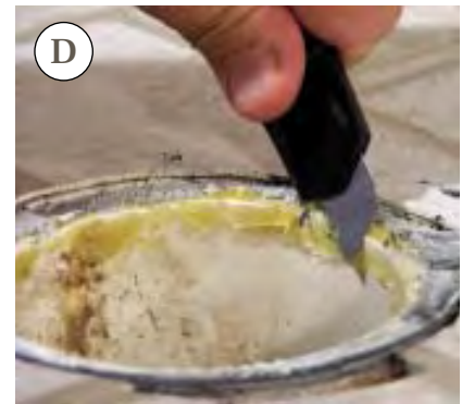
Figure 4. In cases where a closet flange is surface-mounted (rather than flush to the floor), the author slips a simple cable saw (A) under the flange and pulls it back and forth in a sawing motion to cut through the plastic (B). He removes the damaged flange (C), cleans up the cut with a utility knife (D), and then installs a replacement flange that slips inside the existing drainpipe.
