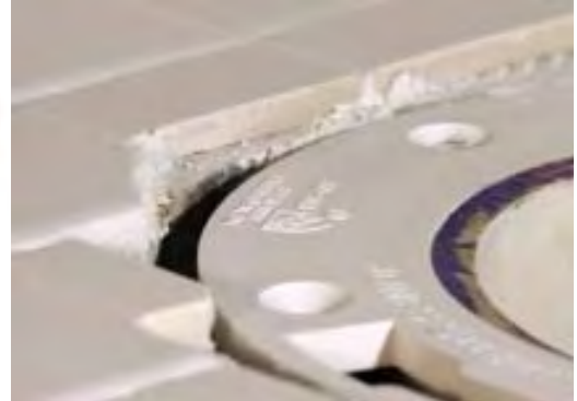
Figure 7. Flange spacers (left) can be used to raise a closet flange installed below the level of the finished floor (above). Multiple spacers are fine, but each must be sealed to the surface below with silicone caulk and securely fastened to the flooring.
