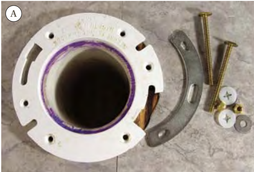
Figure 1. Spanner flanges (A) make repairing broken bolt slots easy. First, the author removes the screws holding the closet flange in place; then he inserts the closet bolt (B). Next, he slides the spanner under the broken portion of the flange (C). While reattaching the closet flange to the floor, he threads some screws through slots in the spanner flange to help hold it in position and strengthen the assembly (D).
