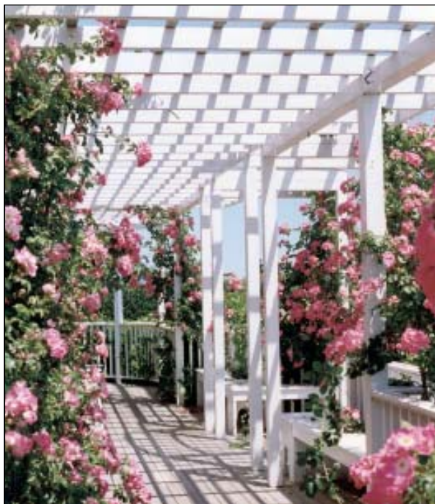
FIGURE 5. A trellis-covered deck provides a natural transition between indoors and out. The deck beneath the trellises was framed conventionally with 2x6 pressure-treated joists, spaced 16 inches on-center, and supported by a spaced ledger against the house and by a 6x6 grade beam on 12-inch-diameter concrete piers around the perimeter. The decking itself is 3/4x4 Doug fir, spaced 1/8 inch apart, nailed to the joists with stainless-steel ring-shank nails.
