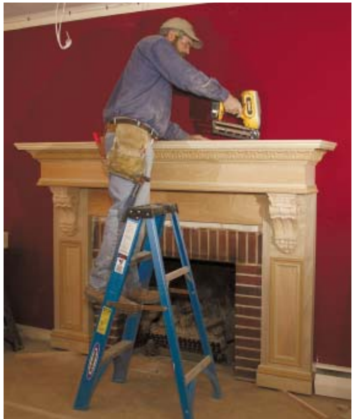
Figure 8. A horizontal cleat (above) provides nailing for the box mantelshelf, which is installed after the lower pilasters (right).
