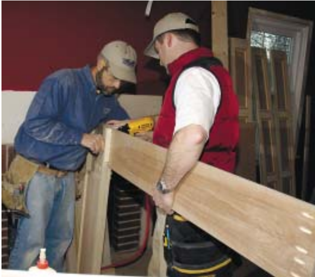
Figure 7. To help ensure that the assembly will be plumb and level, the author pins and then pocket-screws the lower pilasters to the plywood frieze before installing them (left). MDF cleats glued and nailed to the wall provide secure fastening for the pilasters (right).
