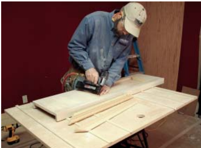
Figure 3. The pilaster panels are trimmed out with an imprinted panel molding. To help size the panels so that the pattern remains continuous as it turns the corners (top), the author lays out the stiles and rails using a precut section of molding as a spacing jig (center). He back-cuts the miters slightly with a block plane so they'll slip easily into place during installation (above).
