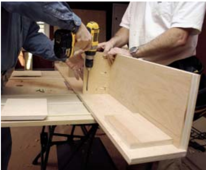
Figure 5. The mantelshelf begins as a plywood box, butt-jointed along the bottom edge and with the front and sides mitered together. A few cleats pocket-screwed inside reinforce the box (above); the butt joint is covered with molding (right).
