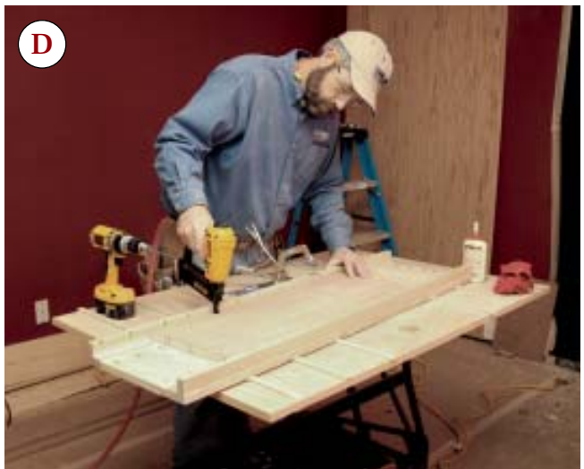
Figure 2. Because pocket-screw joints go together quickly and require little clamping or sanding, the author uses them to build the frame-and-panel assemblies that make up the mantel (A). To add depth to the pilasters, he glues and pocket-screws 1-by rippings to the frames, pinning them in place first so that they are inset slightly from the edges of the panel (B); later, he will trim the panel edges flush with a router (C). Next, after fastening the plywood panel to the frame (D), he fills in voids and dings with wood glue mixed with sawdust, then cleans up the joinery with a few passes of a belt sander (E).
