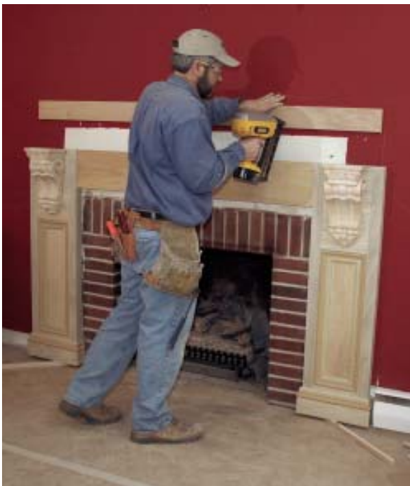
Figure 8. A horizontal cleat (above) provides nailing for the box mantelshelf, which is installed after the lower pilasters (right).
