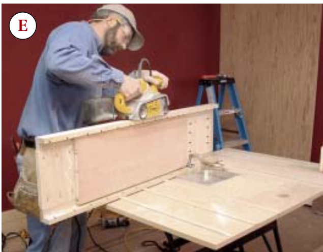
Figure 2. Because pocket-screw joints go together quickly and require little clamping or sanding, the author uses them to build the frame-and-panel assemblies that make up the mantel (A). To add depth to the pilasters, he glues and pocket-screws 1-by rippings to the frames, pinning them in place first so that they are inset slightly from the edges of the panel (B); later, he will trim the panel edges flush with a router (C). Next, after fastening the plywood panel to the frame (D), he fills in voids and dings with wood glue mixed with sawdust, then cleans up the joinery with a few passes of a belt sander (E).
