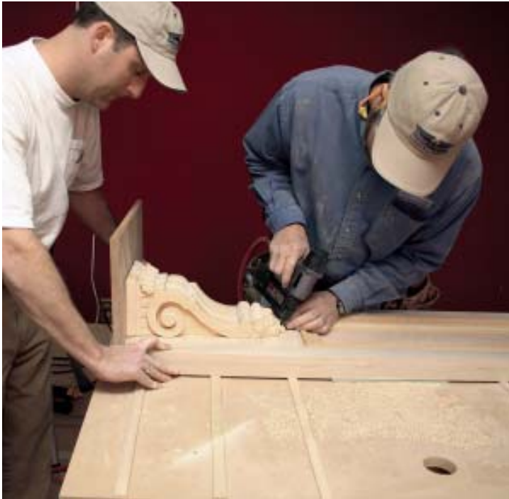
Figure 4. After applying glue and carefully positioning the corbels, the author pins each in place to make sure it won't move, then screws into it through the back of the panel for a strong connection (left). When installing the pilaster bases, he is careful to place the molding so that the repeating pattern turns the mitered corners symmetrically (above).
