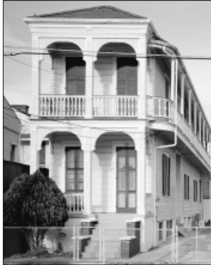
The early “shotgun” homes (above) of New Orleans (so-called because they had no hallways and each room opened into the next all the way through the house), were built on piers at least 3 feet high in anticipation of flooding, and they traditionally included wind-resistant hip roofs.
