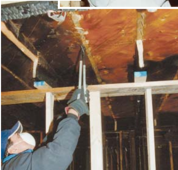
Figure 6. To replace burned floor joists without damaging the finish floor, the author's crew first builds temporary shoring to support the floor system (above). After damaged joist sections have been cut off with a reciprocating saw and removed with a pry bar (right), a worker clips off nails from underneath so that new joists can be installed without damage to the finish flooring above (below).
