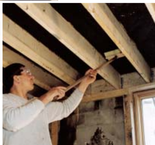
Figure 11. A simple pump-sprayer is an effective way to saturate smoke-damaged areas with detergents, solvents, and deodorants (above). To help eliminate smoky odors, these exposed and charred — but structurally sound — joists are given a final scrubbing (right).
