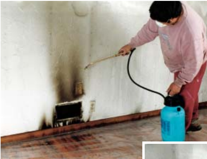
Figure 12. Because heat causes paints to become porous, household cleansers tend to smear rather than remove dirt; specialty cleansers that combine solvents and detergents are more effective and can also be fortified with odor-fighting additives. A pump-sprayer is an effective way to apply the cleaner (above), but sometimes there is no substitute for elbow grease (right). After cleaning, spraying a soot sealer on the walls with an airless paint sprayer locks in any residual odors before the walls are primed and repainted (below).
