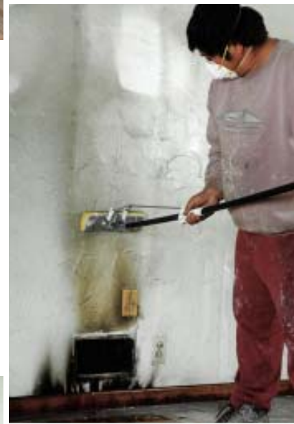
Figure 12. Because heat causes paints to become porous, household cleansers tend to smear rather than remove dirt; specialty cleansers that combine solvents and detergents are more effective and can also be fortified with odor-fighting additives. A pump-sprayer is an effective way to apply the cleaner (above), but sometimes there is no substitute for elbow grease (right). After cleaning, spraying a soot sealer on the walls with an airless paint sprayer locks in any residual odors before the walls are primed and repainted (below).
