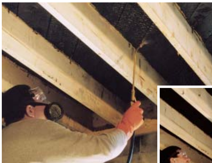
Figure 11. A simple pump-sprayer is an effective way to saturate smoke-damaged areas with detergents, solvents, and deodorants (above). To help eliminate smoky odors, these exposed and charred — but structurally sound — joists are given a final scrubbing (right).
