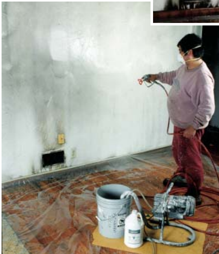
Figure 12. Because heat causes paints to become porous, household cleansers tend to smear rather than remove dirt; specialty cleansers that combine solvents and detergents are more effective and can also be fortified with odor-fighting additives. A pump-sprayer is an effective way to apply the cleaner (above), but sometimes there is no substitute for elbow grease (right). After cleaning, spraying a soot sealer on the walls with an airless paint sprayer locks in any residual odors before the walls are primed and repainted (below).
