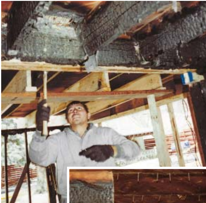
Figure 6. To replace burned floor joists without damaging the finish floor, the author's crew first builds temporary shoring to support the floor system (above). After damaged joist sections have been cut off with a reciprocating saw and removed with a pry bar (right), a worker clips off nails from underneath so that new joists can be installed without damage to the finish flooring above (below).
