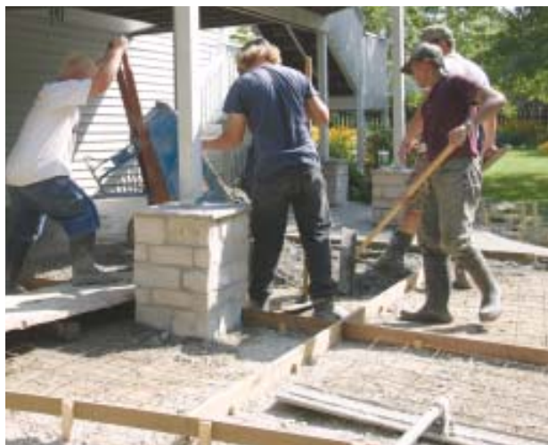
Figure 6. These cedar control joints divide the slab into sections that can be poured one at a time.
