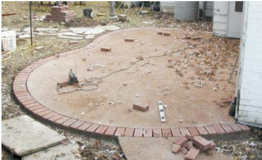
Figure 12. At left, the author's crew cuts stone to form an inset medallion in an aggregate finish driveway. Below, a brick head course set into a patio waits to be grouted.
