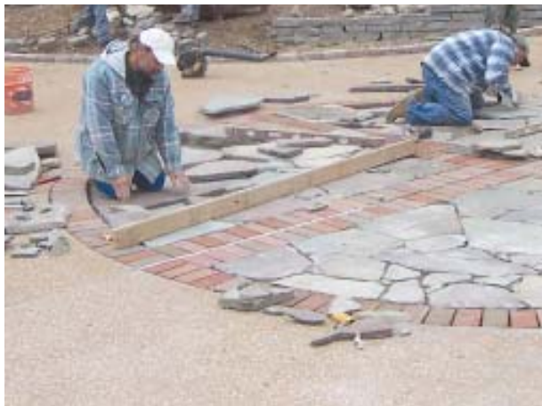
Figure 12. At left, the author's crew cuts stone to form an inset medallion in an aggregate finish driveway. Below, a brick head course set into a patio waits to be grouted.
