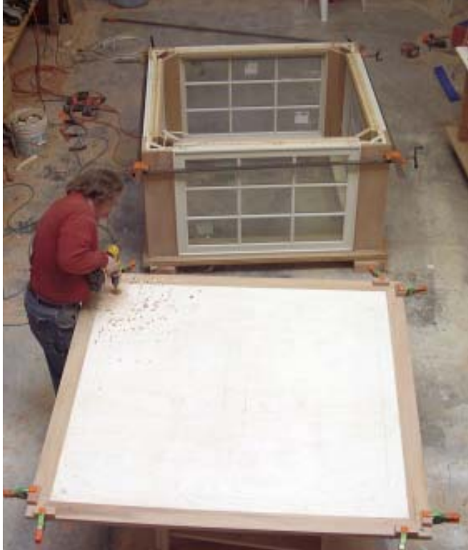
Figure 4. A carpenter drills a hole in the ceiling panel for a light fixture (left). Clamped-on corner blocks will help guide the ceiling panel into exact position. A simple full-scale stick pattern of the roof (above) provides exact dimensions and cut angles for the hips and soffit details.
