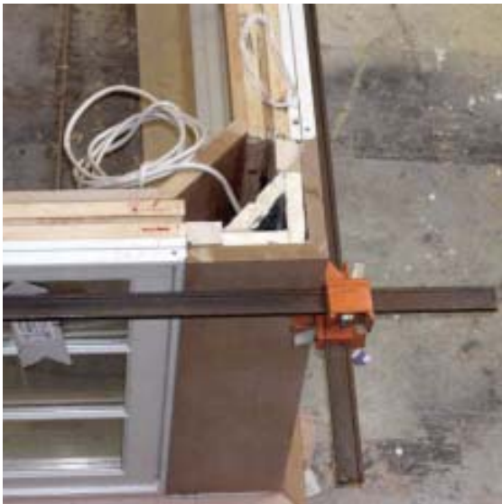
Figure 3. Metal-clad awning windows were screwed from beneath to the plywood base (above). Mitered cedar corner boards were joined with two-part epoxy, then attached to blocks at the window edges (above left). A triangular support on the inside runs the height of each corner (left). A length of 14-3 wire was provided for an eventual ceiling fan or light fixture; a nylon pull string stands by should additional wiring be needed.
