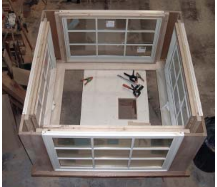
Figure 3. Metal-clad awning windows were screwed from beneath to the plywood base (above). Mitered cedar corner boards were joined with two-part epoxy, then attached to blocks at the window edges (above left). A triangular support on the inside runs the height of each corner (left). A length of 14-3 wire was provided for an eventual ceiling fan or light fixture; a nylon pull string stands by should additional wiring be needed.
