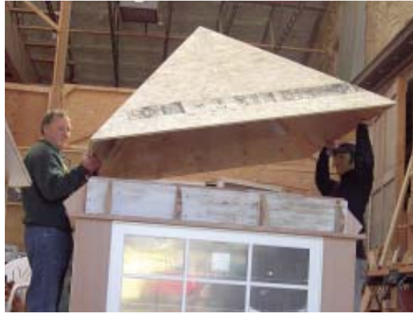
Figure 6. Lookout blocks installed against a 5/4 backer board will support the crown molding (left). Square-cut blocks behind the backer hold it perfectly plumb. Two-inch-thick rigid foam board provides a measure of ceiling insulation. The completed cone assembly was dry-fit (above) before being glued and screwed into place.
