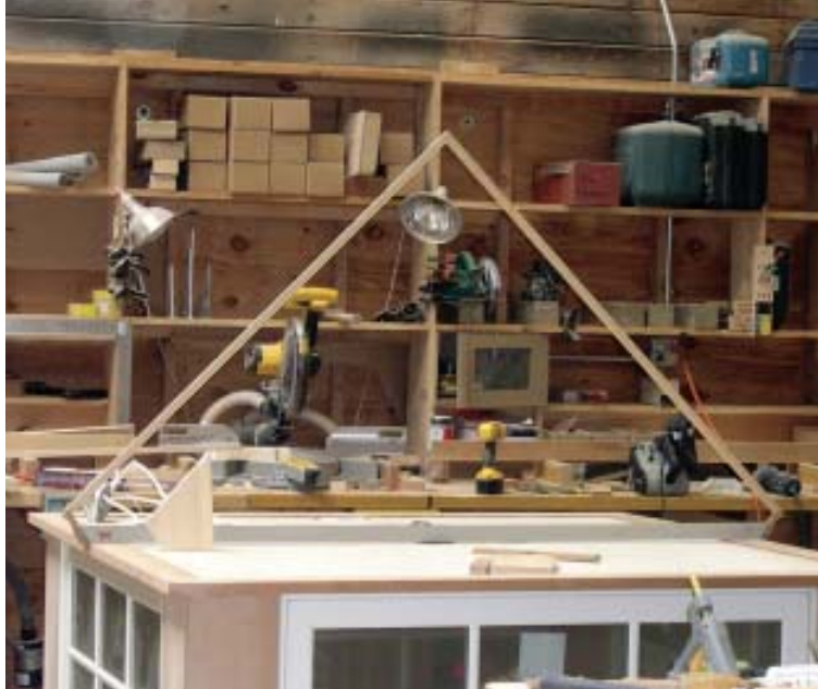
Figure 4. A carpenter drills a hole in the ceiling panel for a light fixture (left). Clamped-on corner blocks will help guide the ceiling panel into exact position. A simple full-scale stick pattern of the roof (above) provides exact dimensions and cut angles for the hips and soffit details.
