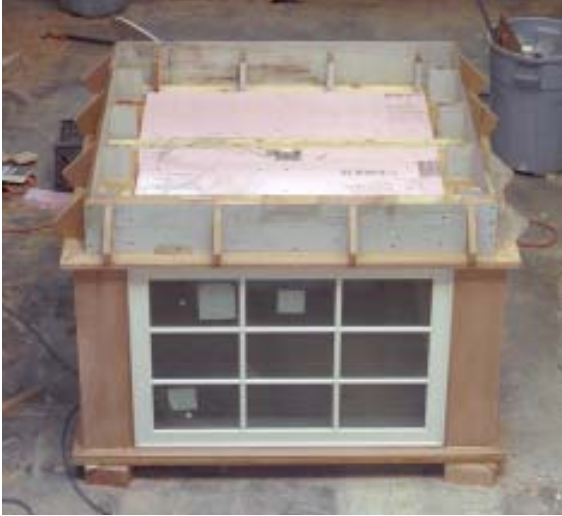
Figure 6. Lookout blocks installed against a 5/4 backer board will support the crown molding (left). Square-cut blocks behind the backer hold it perfectly plumb. Two-inch-thick rigid foam board provides a measure of ceiling insulation. The completed cone assembly was dry-fit (above) before being glued and screwed into place.
