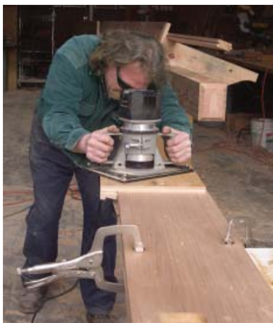
Figure 2. Following the shape of the band-sawn rafter tail, the author used a bottom-bearing bit (above) to profile the end of the attached rake frieze (right), which was glued to the tail with two-part epoxy. Once in place, the rake board looks like a full-dimension timber rafter (far right).
