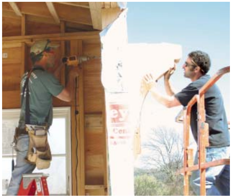
Figure 9. After wrestling the knee bracket into place on temporary supports (left), one carpenter stabilized it (below, left) while the other attached it with lag screws through the framing inside (below).
