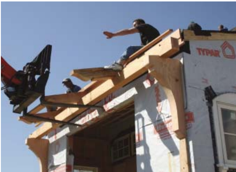
Figure 10. Resting on shop dollies, the 42-foot beam and rafter-tail assembly awaited transport to the site (left, top). On site, the heavy lifting was done by a material handler as a carpenter guided the assembly into place on the knee brackets (above and right).
