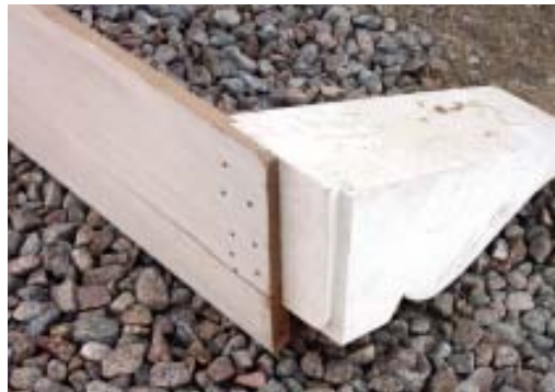
Figure 5. The stub tenons used to attach the tails to the frieze are stepped in so that any shrinkage of the tail does not leave an unsightly gap in the joint (left). Structural screws hold the tails to the 5/4 frieze board; any butt joints are mostly concealed behind the corbels (above).
