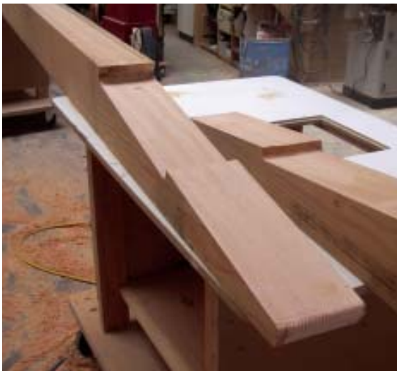
Figure 7. To make a 42-foot-long carrying beam, the author joined two pieces with a locking scarf joint, using the same router template to cut the identical profiles (left). The two pieces are forced tightly together by a pair of opposing wedges at the joint's center (above). While such lap joints are strong even when assembled dry, the author applied two-part epoxy to prevent water entry and further increase the joint's strength.
