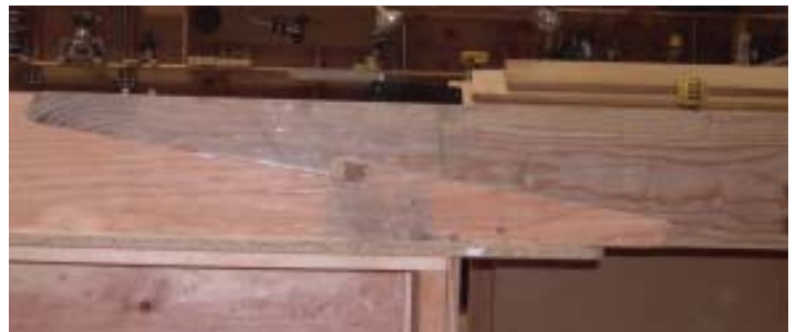
Figure 7. To make a 42-foot-long carrying beam, the author joined two pieces with a locking scarf joint, using the same router template to cut the identical profiles (left). The two pieces are forced tightly together by a pair of opposing wedges at the joint's center (above). While such lap joints are strong even when assembled dry, the author applied two-part epoxy to prevent water entry and further increase the joint's strength.
