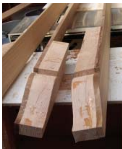
Figure 2. Following the shape of the band-sawn rafter tail, the author used a bottom-bearing bit (above) to profile the end of the attached rake frieze (right), which was glued to the tail with two-part epoxy. Once in place, the rake board looks like a full-dimension timber rafter (far right).
