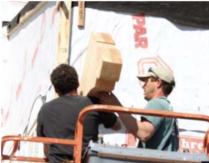
Figure 9. After wrestling the knee bracket into place on temporary supports (left), one carpenter stabilized it (below, left) while the other attached it with lag screws through the framing inside (below).
