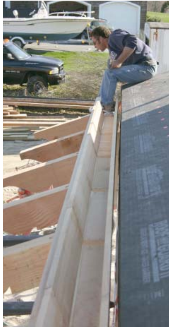
Figure 10. Resting on shop dollies, the 42-foot beam and rafter-tail assembly awaited transport to the site (left, top). On site, the heavy lifting was done by a material handler as a carpenter guided the assembly into place on the knee brackets (above and right).
