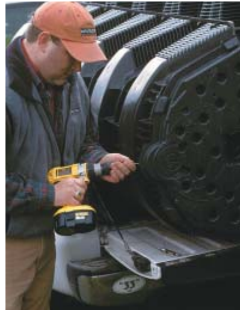
Figure 2. Chamber sections are designed to lock together easily. End caps are installed before placing the sections in the trench. They're molded with the pipe locations, so they can be used at either end of the trench. A couple of galvanized screws hold the end cap in place (right).
