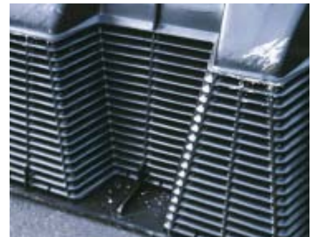
Figure 3. After covering the chambers with sand, the author walks the trenches to make sure nothing has been dislocated and to compact the sand (left). The chamber louvers are sloped so as not to get clogged with fine particles of soil or sand (above).
