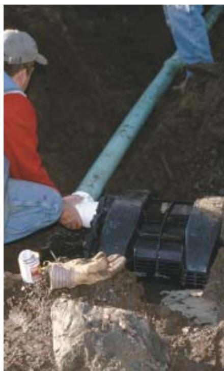
Figure 5. Starting at the box, we work back to the connections on the chambers. The opening in the end cap is drilled with a 4-inch hole. Fittings are attached using PVC cement, and the pipe is cut with a hand saw. Careful backfilling with sand prevents the connections from loosening.
