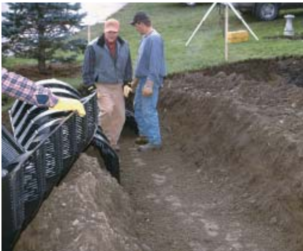
Figure 1. Plastic leach chambers are lightweight and stackable, so they can be delivered to the job in a pickup, making them a good option for sites with poor access. Size vary: These chambers are about 6 feet long and weigh about 40 pounds each. The author places a couple of inches of sand in the trench (right) to make leveling the chambers easier.
