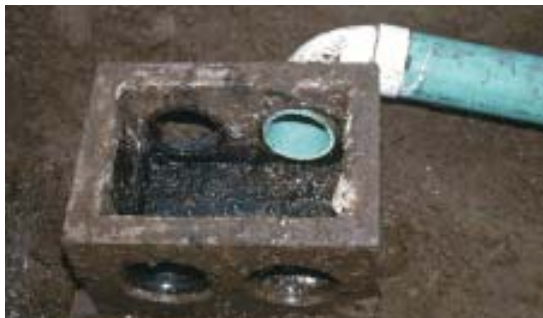
Figure 4. The concrete distribution box divides the effluent equally among the three trenches, so it has to be level. Self-sealing plastic knockouts are used to bring the pipes in and out. Once the connections are made, the cover will be installed and the box carefully backfilled.
