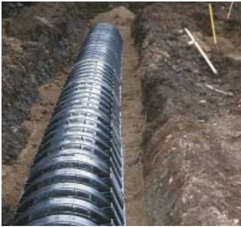
Figure 2. Chamber sections are designed to lock together easily. End caps are installed before placing the sections in the trench. They're molded with the pipe locations, so they can be used at either end of the trench. A couple of galvanized screws hold the end cap in place (right).
