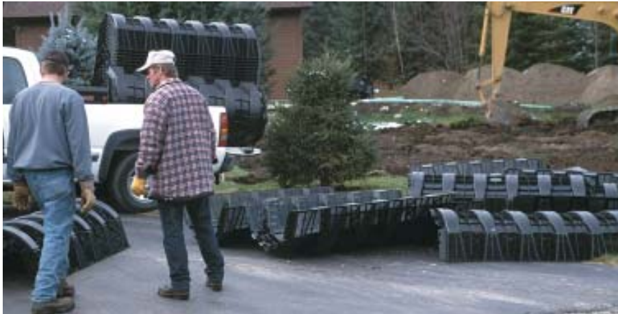
Figure 1. Plastic leach chambers are lightweight and stackable, so they can be delivered to the job in a pickup, making them a good option for sites with poor access. Size vary: These chambers are about 6 feet long and weigh about 40 pounds each. The author places a couple of inches of sand in the trench (right) to make leveling the chambers easier.
