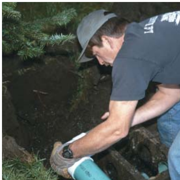
Figure 4. The concrete distribution box divides the effluent equally among the three trenches, so it has to be level. Self-sealing plastic knockouts are used to bring the pipes in and out. Once the connections are made, the cover will be installed and the box carefully backfilled.
