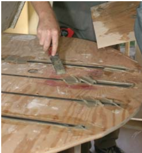
Figure 3. Here, the installer applies epoxy to steel angles in the subtop that will support an overhanging section of counter (left). Another way to stiffen the overhang is to support it from underneath. This section of the subtop (below) is carried by steel plates that span the top of the cabinet.
