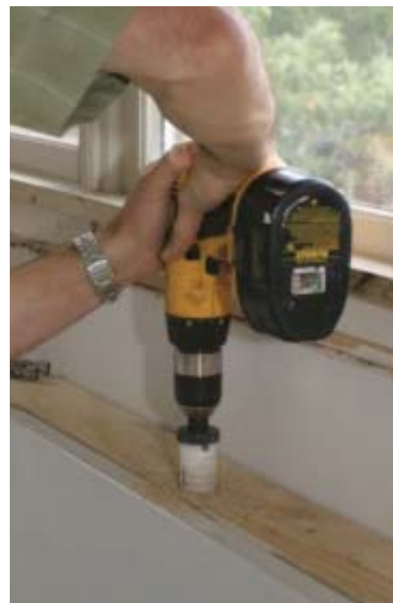
Figure 9. Sinks and faucets must be located and temporarily installed in the subtop before the templates for the counter are made (above left and right). Here, the author is verifying that the homeowner is satisfied with the location of the faucet (left).
