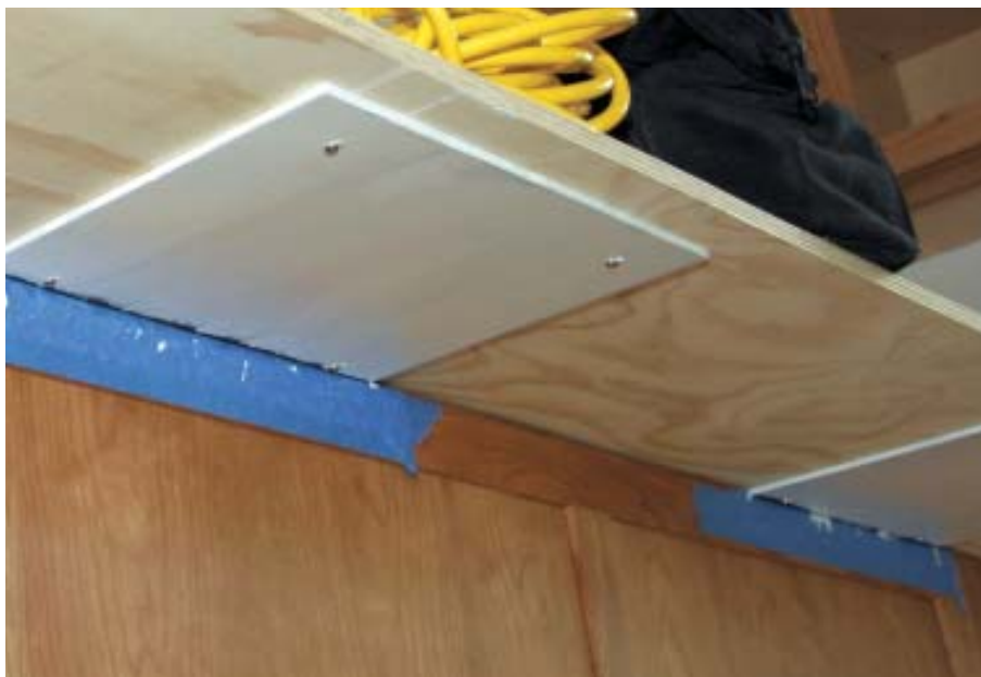
Figure 3. Here, the installer applies epoxy to steel angles in the subtop that will support an overhanging section of counter (left). Another way to stiffen the overhang is to support it from underneath. This section of the subtop (below) is carried by steel plates that span the top of the cabinet.
