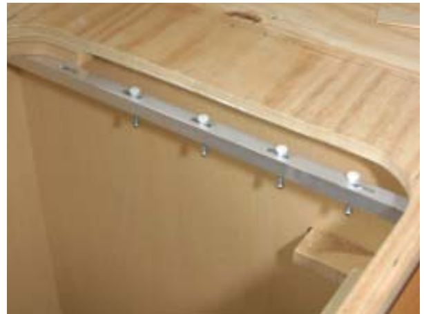
Figure 5. Undermount sinks are supported from underneath the rim. In this kitchen, the front and back edges of the sink will be carried by the lip that is formed between the stretcher and the plywood subtop. Each end will be carried by an adjustable metal bracket (right).
