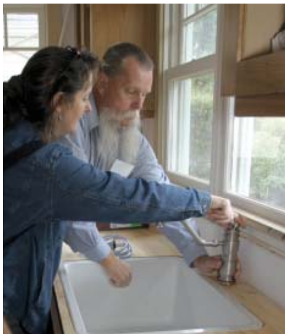
Figure 9. Sinks and faucets must be located and temporarily installed in the subtop before the templates for the counter are made (above left and right). Here, the author is verifying that the homeowner is satisfied with the location of the faucet (left).
