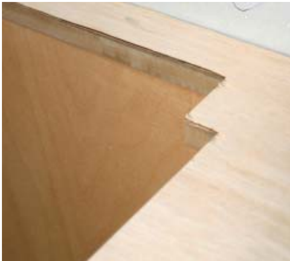
Figure 10. The top piece is a 1/8-inch plywood template that has been cut to match the opening in the subtop for a cooktop and downdraft vent. The vent is not as wide as the cooktop, which is why the opening is narrower at the back.
