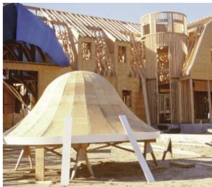
Figure 10. One section of the roof sheathing was left off to allow for access inside the tower for installation (right). The roof was finished with a bendable plastic fascia and cedar shingles (below).
