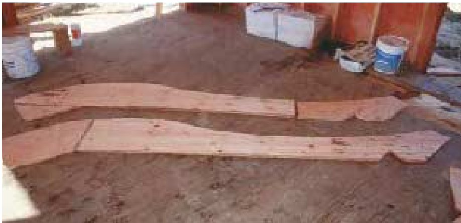
Figure 6. Double-layer rafters, glued and nailed together with staggered joints, were laid out with trammel sticks on the deck.
