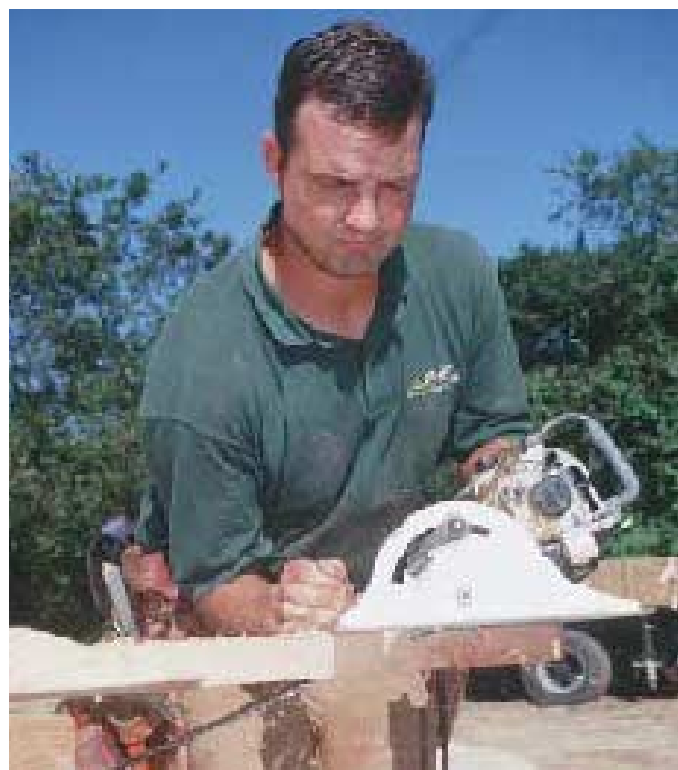
Figure 8. The author determined the bevel cuts for the rafters (right) by drawing a full-size overhead plan view on plywood, then cut the acute angles with a modified wormdrive saw mounted on a swing-table adapter (below).
