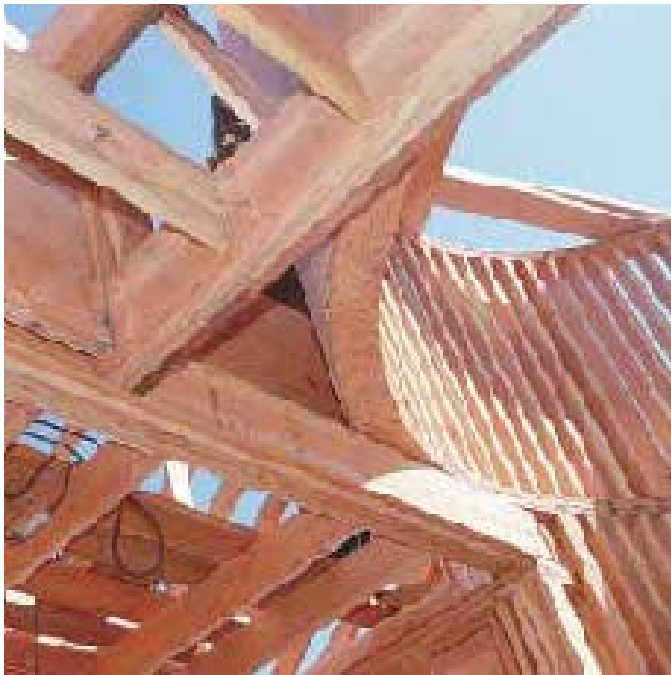
Figure 3. The top, full-round section of the tower was framed on the ground and hoisted into place with a material lift (top). The round section dropped neatly into place in a square opening framed to support it (above and right).
