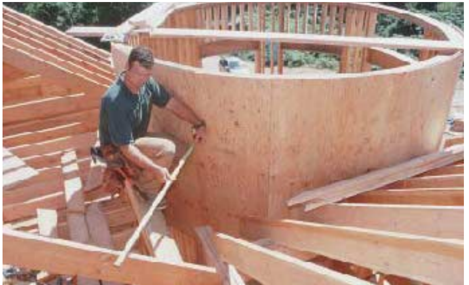
Figure 5. Plywood bends more easily parallel to the face grain, so the carpenters installed the double-layer \frac{3}{8} -inch sheathing vertically (above). A lip at the top of the tower wall captured the bottom plate of the roof (above right). At right, the author measures for a cricket where the tower interrupts a valley.
