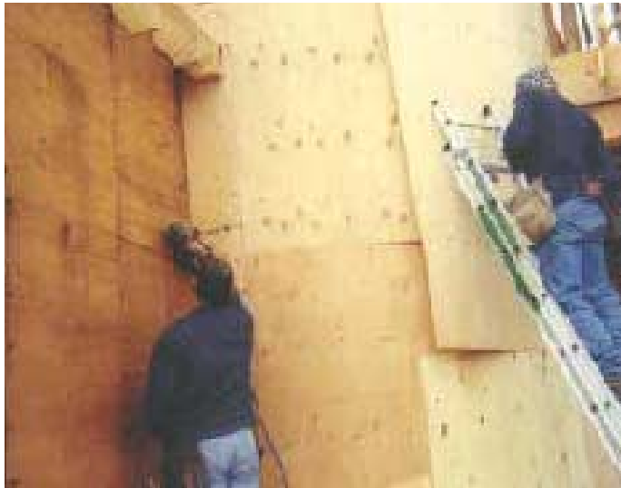
Figure 5. Plywood bends more easily parallel to the face grain, so the carpenters installed the double-layer \frac{3}{8} -inch sheathing vertically (above). A lip at the top of the tower wall captured the bottom plate of the roof (above right). At right, the author measures for a cricket where the tower interrupts a valley.
