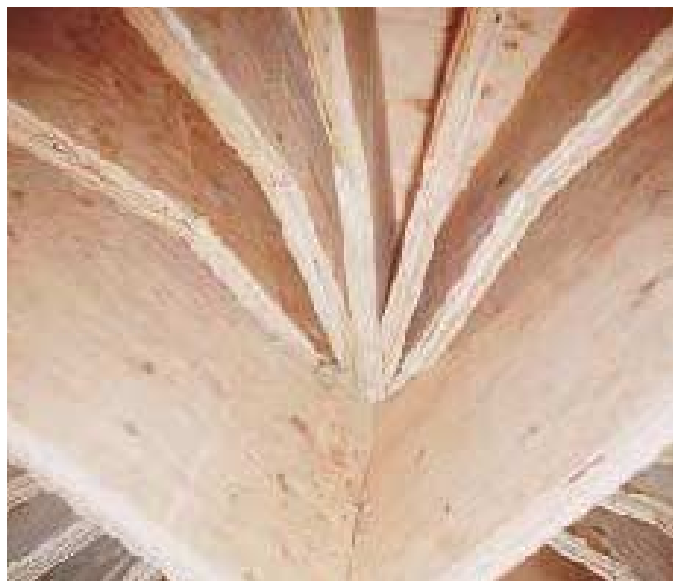
Figure 8. The author determined the bevel cuts for the rafters (right) by drawing a full-size overhead plan view on plywood, then cut the acute angles with a modified wormdrive saw mounted on a swing-table adapter (below).
