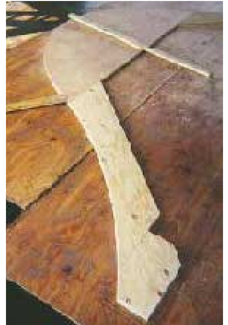
Figure 6. Double-layer rafters, glued and nailed together with staggered joints, were laid out with trammel sticks on the deck.
