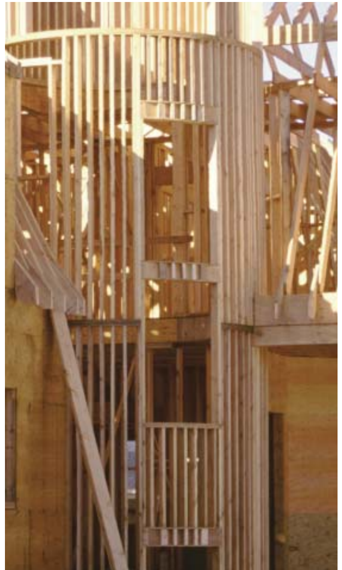
Figure 4. Simple curved window headers were made with doubled 2x8s sandwiched between plywood plate segments (left). Cripple blocking was added on the outside face where needed (below).
