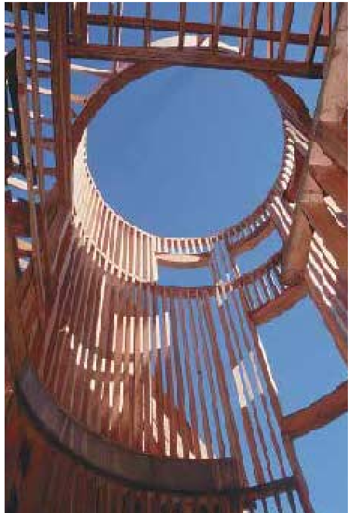
Figure 3. The top, full-round section of the tower was framed on the ground and hoisted into place with a material lift (top). The round section dropped neatly into place in a square opening framed to support it (above and right).
