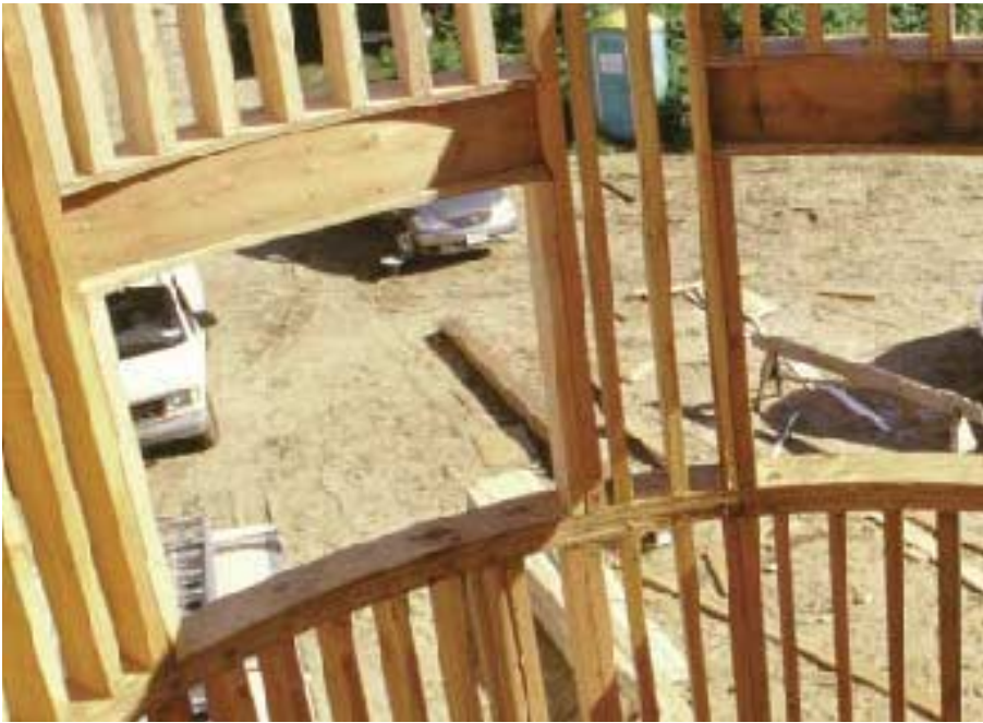
Figure 4. Simple curved window headers were made with doubled 2x8s sandwiched between plywood plate segments (left). Cripple blocking was added on the outside face where needed (below).
