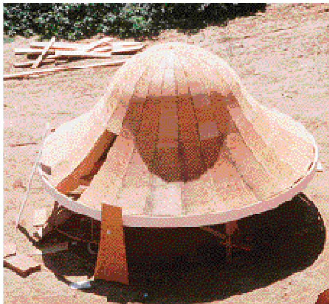
Figure 10. One section of the roof sheathing was left off to allow for access inside the tower for installation (right). The roof was finished with a bendable plastic fascia and cedar shingles (below).
