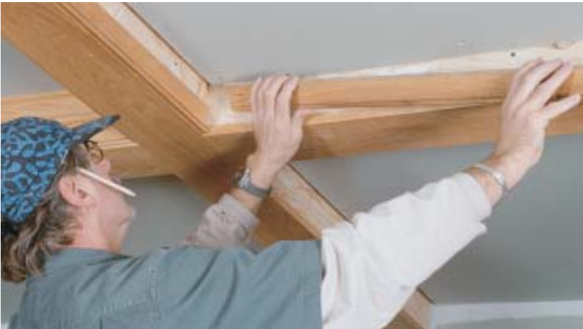
Figure 4. To avoid wasting stock, the side pieces are only as wide as they need to be (left); the crown molding covers the rest (right).
