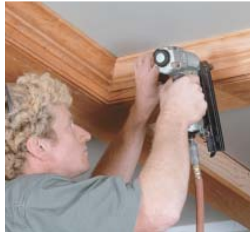
Figure 4. To avoid wasting stock, the side pieces are only as wide as they need to be (left); the crown molding covers the rest (right).
