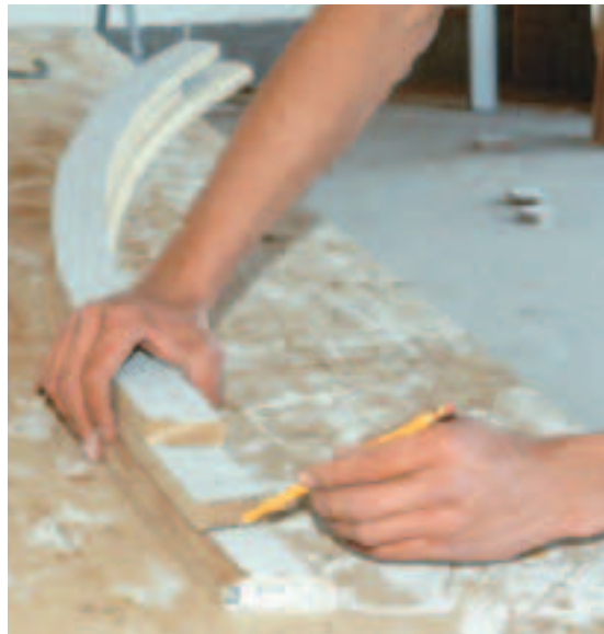
Figure 2. Two extra pieces of railing served as an extendible template for laying out the radius rails (above). After scribing the ends to fit the posts, the carpenters stretched the two pieces apart until they were tight against the new posts, then fastened the pieces together with drywall screws. Tracing the template directly onto the railings guaranteed a tight fit (right).
