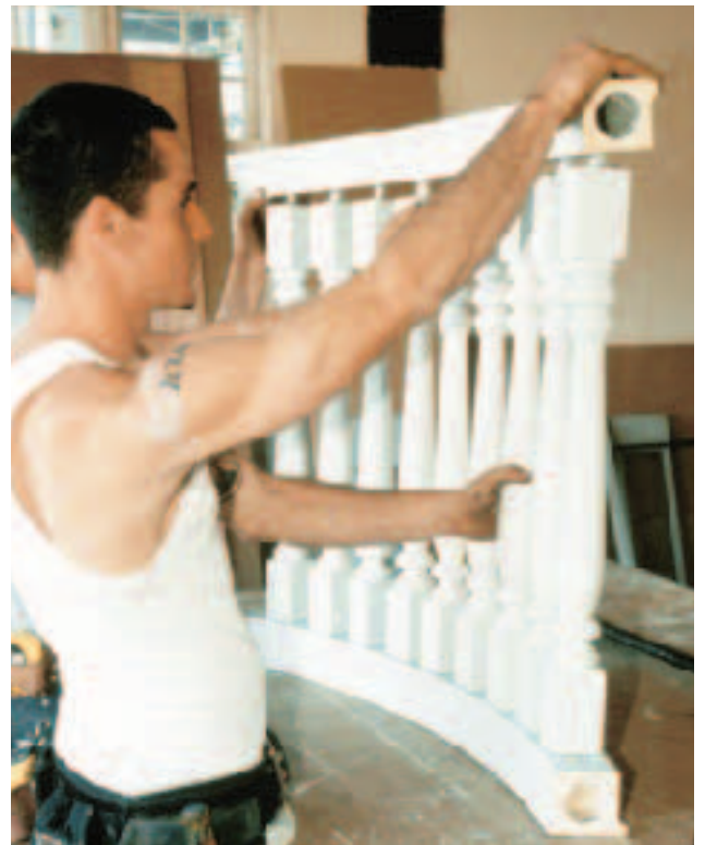
Figure 6. When assembling the Fypon railings (left), 2 1 / 2 -inch galvanized finish nails, four in each baluster, provided temporary security until the polyurethane adhesive dried. Fitting the top rail (above) was tricky and required two sets of hands because of the varying lengths of the 3 / 4 -inch pipe projecting out the end of the balusters. This required finding and setting the longest dowels first.
