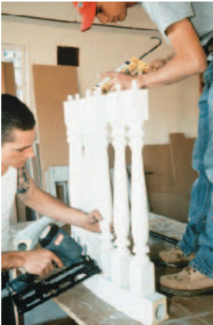
Figure 6. When assembling the Fypon railings (left), 2 1 / 2 -inch galvanized finish nails, four in each baluster, provided temporary security until the polyurethane adhesive dried. Fitting the top rail (above) was tricky and required two sets of hands because of the varying lengths of the 3 / 4 -inch pipe projecting out the end of the balusters. This required finding and setting the longest dowels first.
