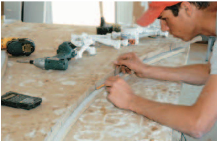
Figure 3. Instead of trying to lay out the spindle centers on the curve, the author used a thin strip of flexible material, marking it in a straight position then bending it to the radius to transfer the marks.
