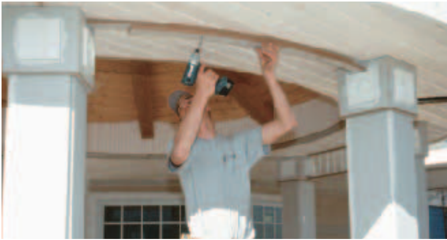
Figure 2. Two extra pieces of railing served as an extendible template for laying out the radius rails (above). After scribing the ends to fit the posts, the carpenters stretched the two pieces apart until they were tight against the new posts, then fastened the pieces together with drywall screws. Tracing the template directly onto the railings guaranteed a tight fit (right).
