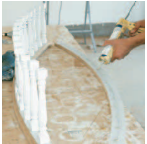
Figure 4. Holes for the galvanized screws were predrilled in both the rail and the spindles (left), but the Fypon adhesive provides the real strength for the spindle assemblies (right).
