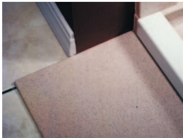
Figure 3. Ramp kits are available when recessing the base isn't feasible.
