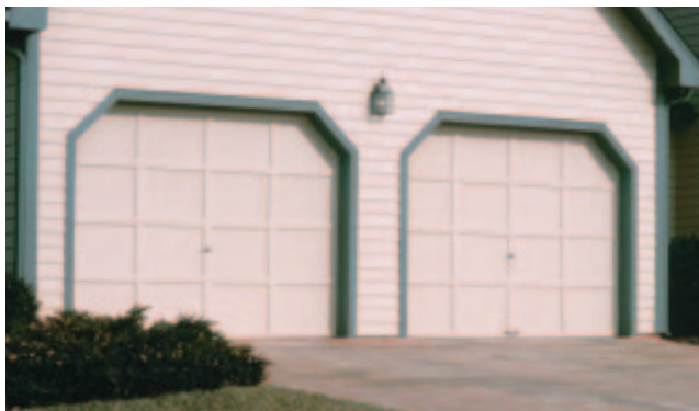
Figure 5. Although steel doors have largely replaced wood-frame doors with hardboard panels, some customers still prefer the crisp appearance of the older style. This simple uninsulated door, made by Amarr, goes for about $360.
