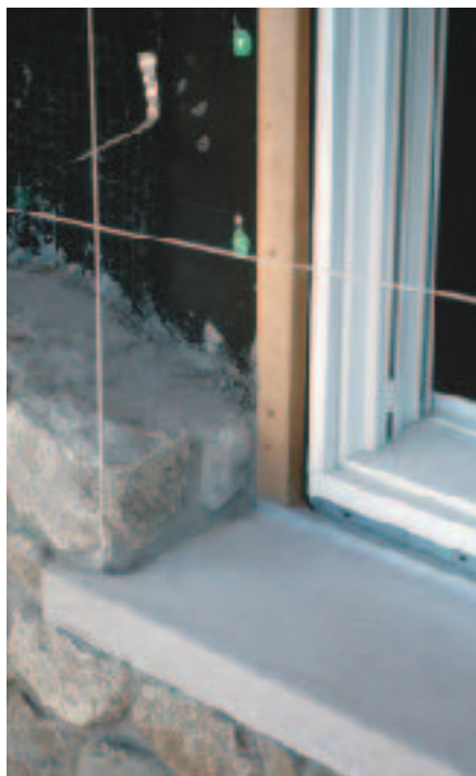
Figure 5. A temporary stick stands in for the window casing during mortar pointing (left). The permanent trim will be bedded in caulk against the cured masonry edge. Stringlines control alignment, and a custom-sawn limestone sill finishes the bottom of the window surround. The author used a section of wood sill molding as a gauge block to position the limestone (above).
