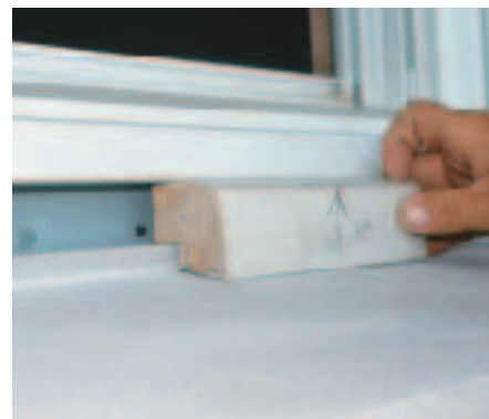
Figure 5. A temporary stick stands in for the window casing during mortar pointing (left). The permanent trim will be bedded in caulk against the cured masonry edge. Stringlines control alignment, and a custom-sawn limestone sill finishes the bottom of the window surround. The author used a section of wood sill molding as a gauge block to position the limestone (above).
