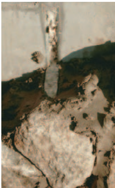
Figure 3. Dovetail channel provides a flexible attachment system over cast concrete (left). The proprietary ties wedge into the channel anywhere along its length (right).
