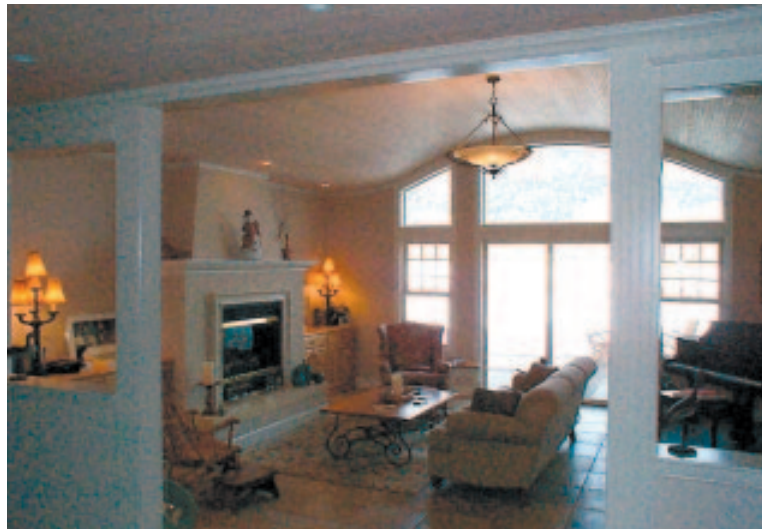
Figure 3. The finished ceiling of beaded fir boards was blind-nailed to blocking sandwiched between the OSB gussets.
