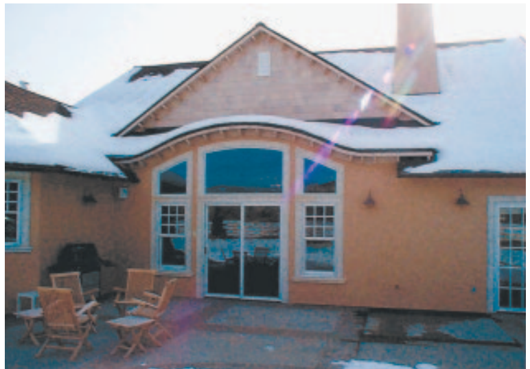
Figure 1. A site-built laminated plywood header defines the eyebrow profile above the patio doors. Short rafters extend from the eyebrow to the peaked roof beyond, which is framed with scissors trusses.
