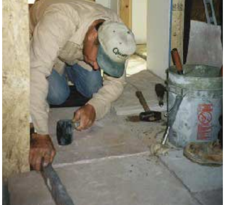
Figure 6. The mason was responsible for cutting in around passages and other obstructions (left). Because the stone was of varying thickness, each piece had to be carefully leveled in reference to the finish floor height (above).
