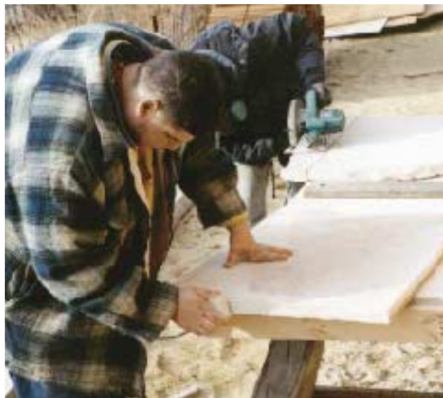
Figure 5. By positioning the kerfed stone slabs (top) on the edge of the table, the workers were able to snap the scored line using a large piece of steel as a hammer (middle). A small scrap of sandstone served to smooth the sharp, rough edges (right).
