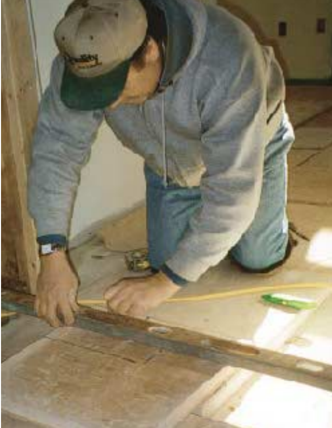
Figure 6. The mason was responsible for cutting in around passages and other obstructions (left). Because the stone was of varying thickness, each piece had to be carefully leveled in reference to the finish floor height (above).
