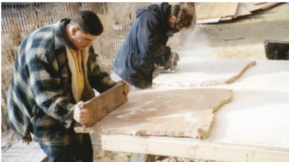
Figure 5. By positioning the kerfed stone slabs (top) on the edge of the table, the workers were able to snap the scored line using a large piece of steel as a hammer (middle). A small scrap of sandstone served to smooth the sharp, rough edges (right).
