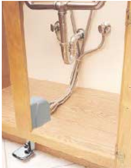
Figure 11. A foot-operable kitchen faucet control keeps greasy hands off the levers.
