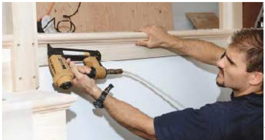
Figure 14. Using 8d nails, the author applies base cap molding around the stringers and landing baseboards. He uses the same material flipped upside down below the stringers on the open side of the stairs, and below the fascia around the open landing.
