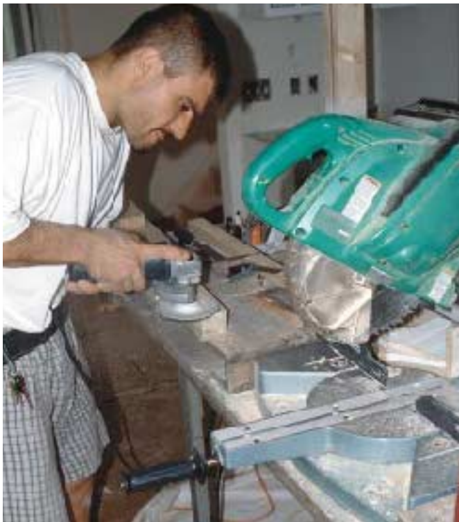
Figure 3. Corner landing posts may be thrown out of plumb or square by the drywall and tape. The author checks for plumb and square (top, left and right), then shims or grinds as needed before attaching the post permanently (above, left and right).
