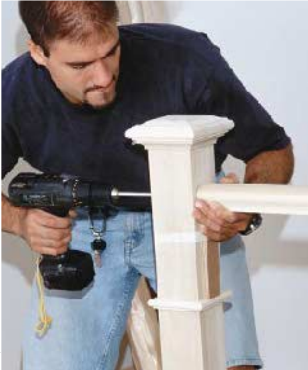
Figure 7. For efficiency and accuracy, the author holds the actual rail in place to mark the cut. Using a measured block to support the rail, he fastens it with screws through the back of the post.
