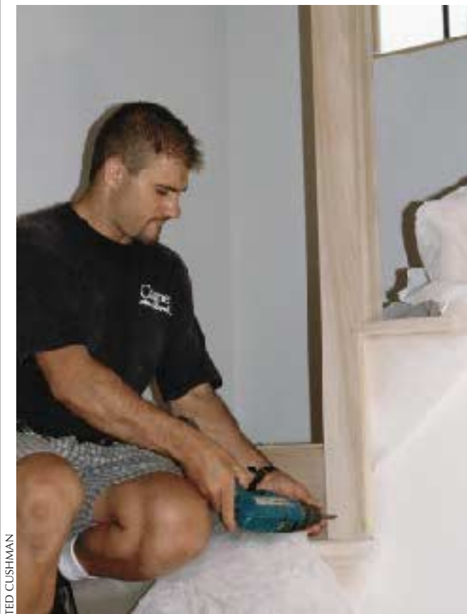
Figure 2. Posts and stair treads are prenotched at the shop to ensure the proper post location and height, but the posts are drilled on site.
