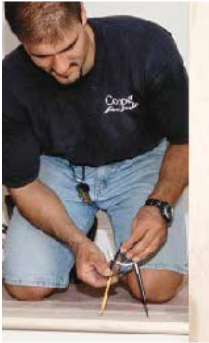
Figure 13. The author marks his hole centers with dividers (left), drills the holes, and transfers the hole centers to a story pole (center), then transfers the same layout onto the underside of the rail (right).
