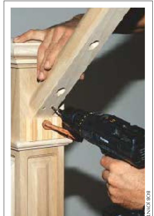
Figure 6. The author uses glue and screws to fasten the rake rail to the post from below. A block clamped to the post steadies it in place.
