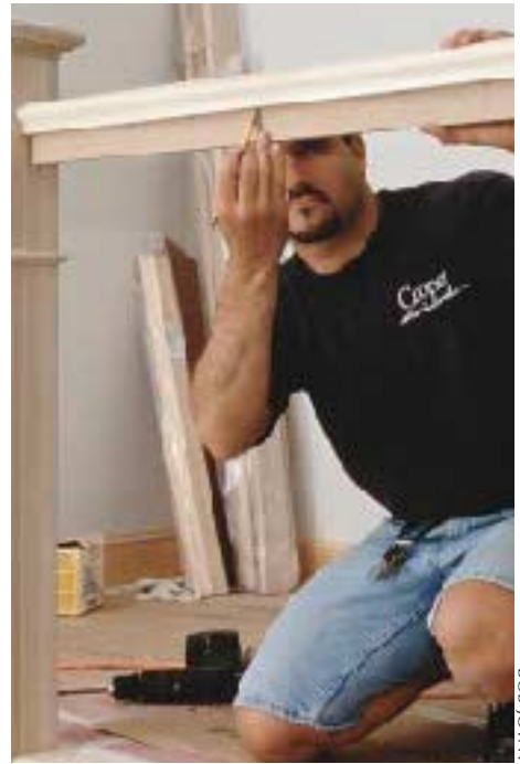
Figure 13. The author marks his hole centers with dividers (left), drills the holes, and transfers the hole centers to a story pole (center), then transfers the same layout onto the underside of the rail (right).
