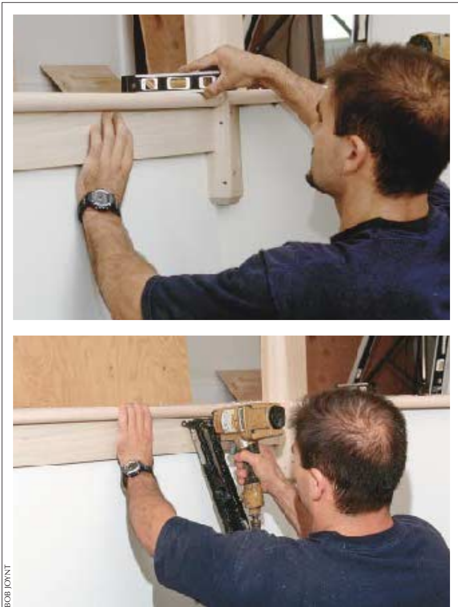
Figure 4. The landing tread helps lock in the newel posts, and hides any shims that may have been used to adjust the post (top). The landing tread must be perfectly level so that no cracks appear at the bottom of the balusters. The author attaches the landing tread with 8d finish nails (above).
