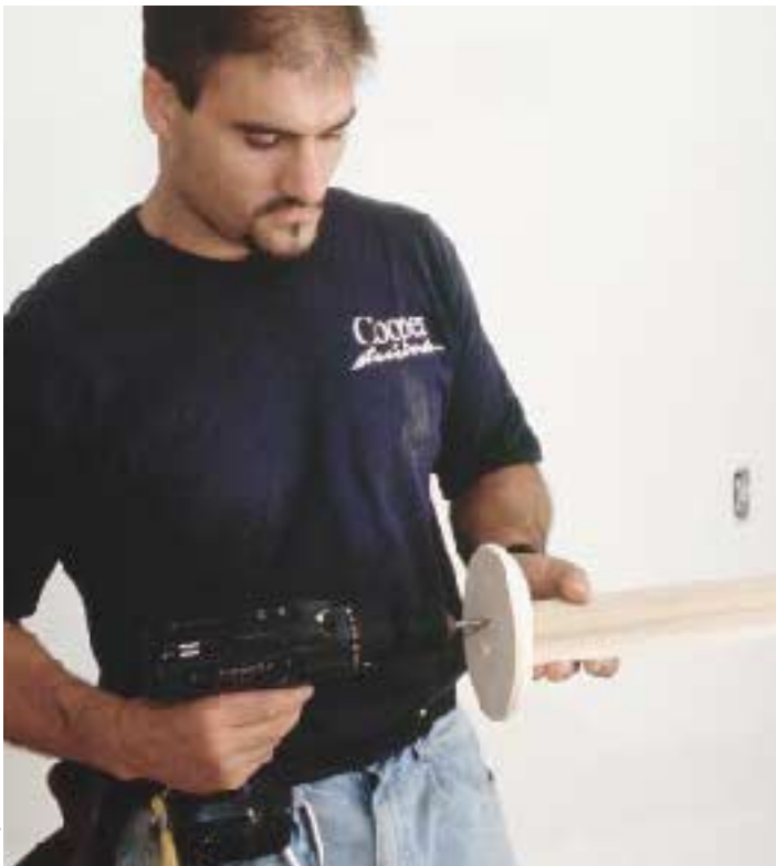
Figure 8. At the wall, the author uses a rosette to attach the rail. He screws the rosette to the end of the rail, then to the wall.
