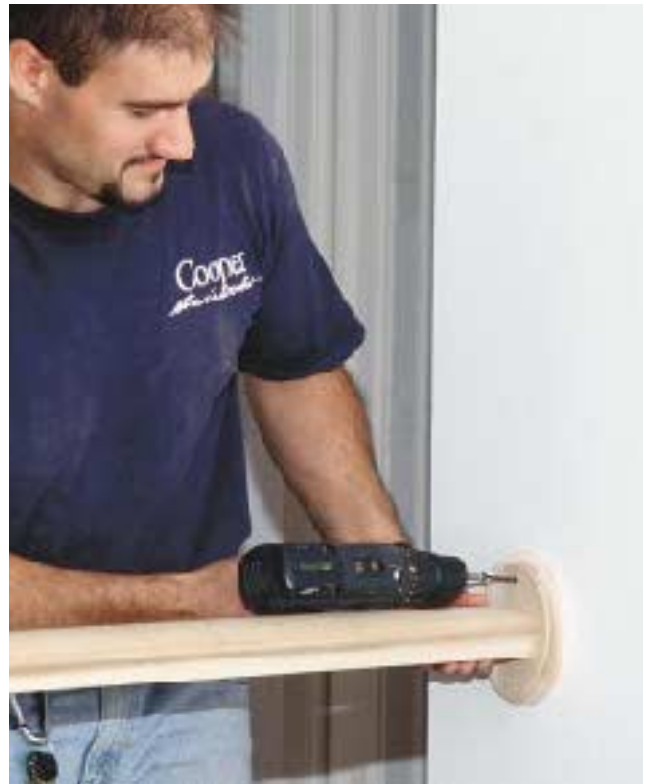
Figure 8. At the wall, the author uses a rosette to attach the rail. He screws the rosette to the end of the rail, then to the wall.
