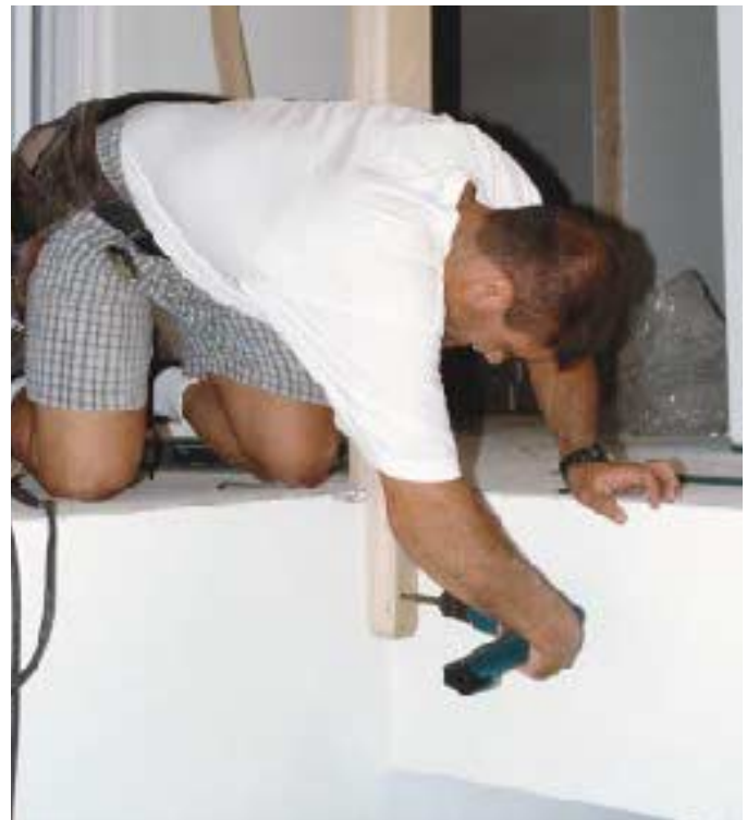
Figure 3. Corner landing posts may be thrown out of plumb or square by the drywall and tape. The author checks for plumb and square (top, left and right), then shims or grinds as needed before attaching the post permanently (above, left and right).
