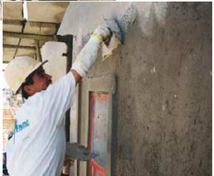
Figure 5. The author's crews pump brown and scratch coats (left). Finish coats (below) are hand-troweled.
