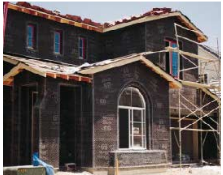
Figure 3. This house is ready for stucco. Special care is taken to ensure the lath is not pulled too tightly at corners. If it is, the stucco will pop off over time. A lath accessory called cornerite (left) can also be used at corners to ensure proper embedment.
