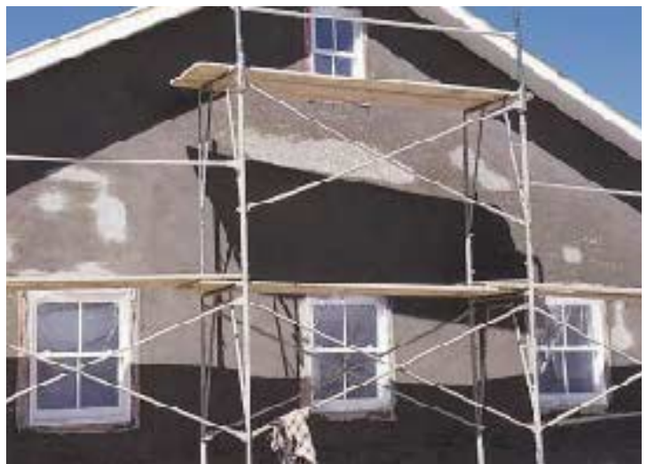
Figure 6. As the scratch coat dries it will change color. It is important to make sure there is enough moisture available for complete hydration of the cement by misting the wall with water.
