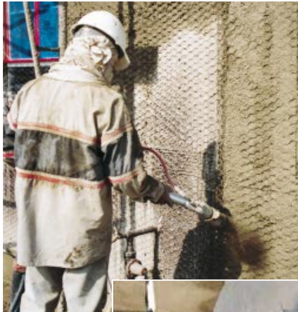
Figure 5. The author's crews pump brown and scratch coats (left). Finish coats (below) are hand-troweled.
