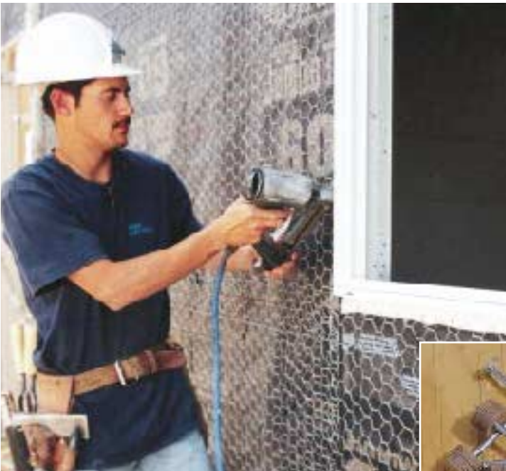
Figure 2. Lath can either be stapled — the fastest method — or nailed. Special furring nails (inset) are designed to hold the lath off the wall so that it's properly embedded in the stucco.
