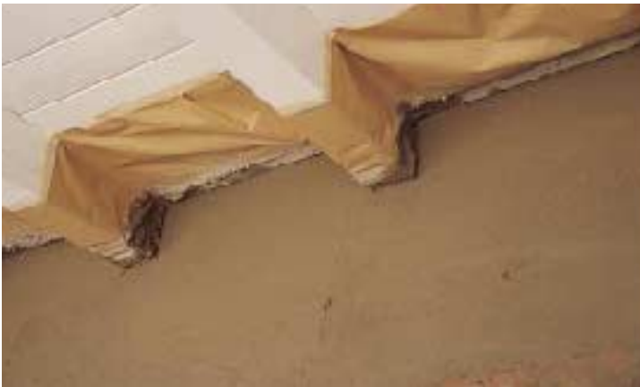
Figure 7. Finish protection is absolutely essential. Make sure you understand who is responsible for this before the job begins.
