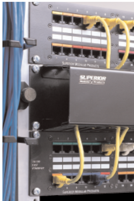
Figure 5. A rack-mount system holds individual punch-down patch panels and distribution blocks, and provides real flexibility for system configuration and expansion. Unlike a recessed panel, it requires dedicated floor space, as in a communications closet.
