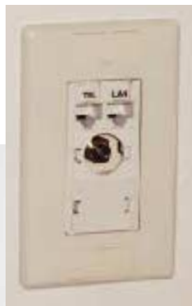
Figure 3. Wire terminals snap into a special faceplate in the "keystone" modular system (left). Other systems employ decorator-style or standard duplex coverplates to unite individual jacks (above).
