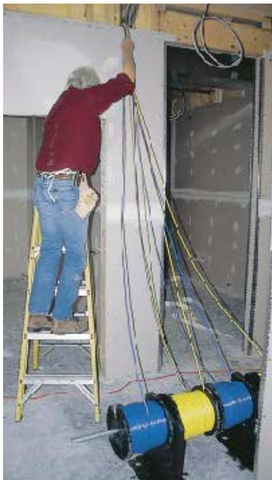
Figure 7. Free-spooling wire is much easier to pay out, and less likely to kink or tangle. A site-built rig is easily made by drilling holes in a couple of studs to hold the spool on a length of pipe.
