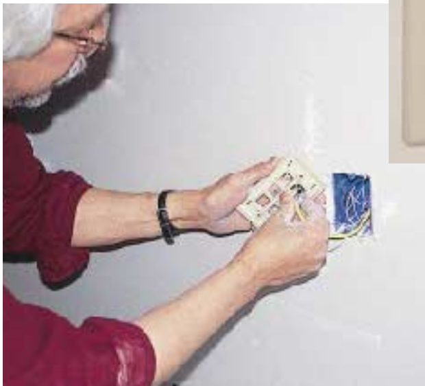
Figure 3. Wire terminals snap into a special faceplate in the "keystone" modular system (left). Other systems employ decorator-style or standard duplex coverplates to unite individual jacks (above).
