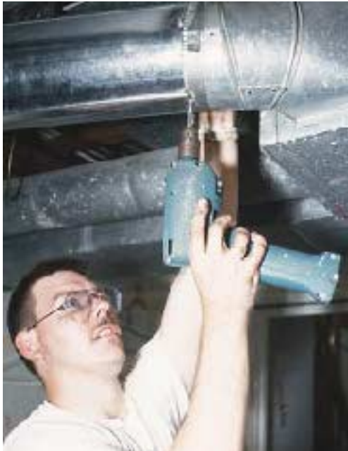
Figure 4. Sheet-metal duct joints must be screwed together before mastic is applied.
