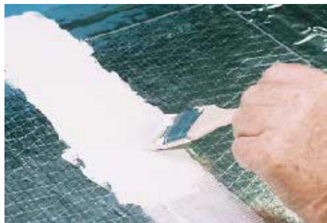
Figure 5. Joints in sheet-metal duct should be sealed with mastic, which can be applied with a paint brush (left). When mastic is used on duct board, the joint should first be bridged with fiberglass tape or scrim (right).
