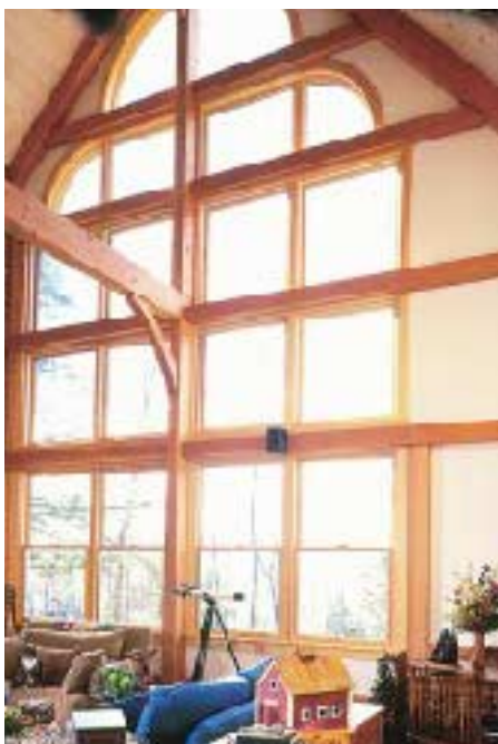
Figure 2. A room with an unusually large area of glass tends to have high heat loss at night and high heat gain on sunny days. Such a room is a good candidate for a separate zone.
