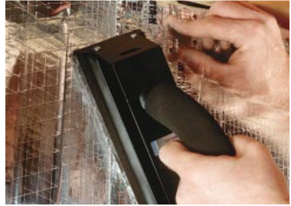
Figure 6. The female end of a duct board joint is pulled taut and stapled through to the male end (left). The joint is completed by applying heat-activated tape, which is warmed with an Amcraft duct board iron (right).
