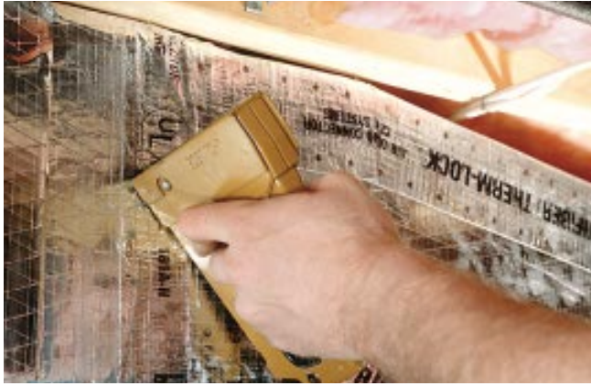
Figure 6. The female end of a duct board joint is pulled taut and stapled through to the male end (left). The joint is completed by applying heat-activated tape, which is warmed with an Amcraft duct board iron (right).
