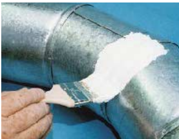
Figure 5. Joints in sheet-metal duct should be sealed with mastic, which can be applied with a paint brush (left). When mastic is used on duct board, the joint should first be bridged with fiberglass tape or scrim (right).
