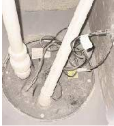
Figure 3. Only the top of the basin shows, allowing service access. Plug-in power simplifies the disconnect.
