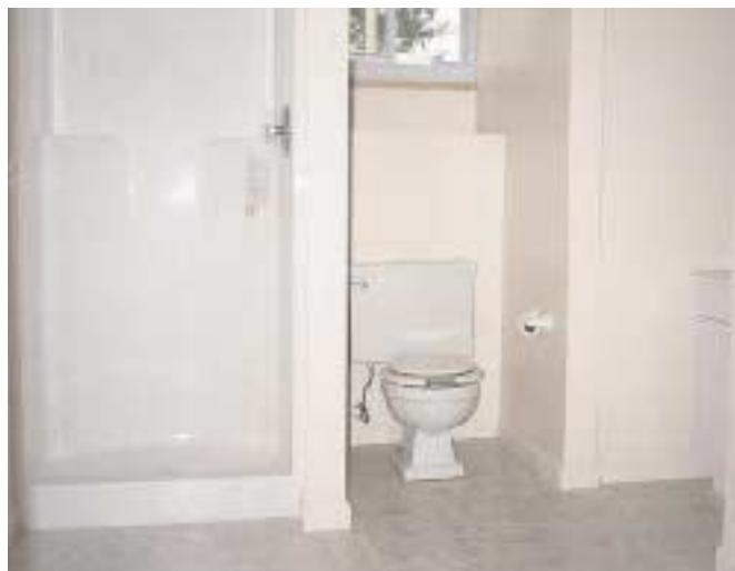
Figure 1. A basement toilet on a platform (above) installs easily but is awkward to use. Using an in-floor basin with a sewage grinder pump creates a normal appearance and doesn't impinge on headroom (right).
