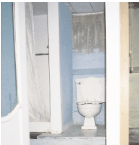
Figure 1. A basement toilet on a platform (above) installs easily but is awkward to use. Using an in-floor basin with a sewage grinder pump creates a normal appearance and doesn't impinge on headroom (right).
