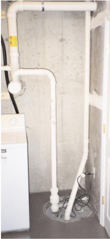
Figure 3. Only the top of the basin shows, allowing service access. Plug-in power simplifies the disconnect.
