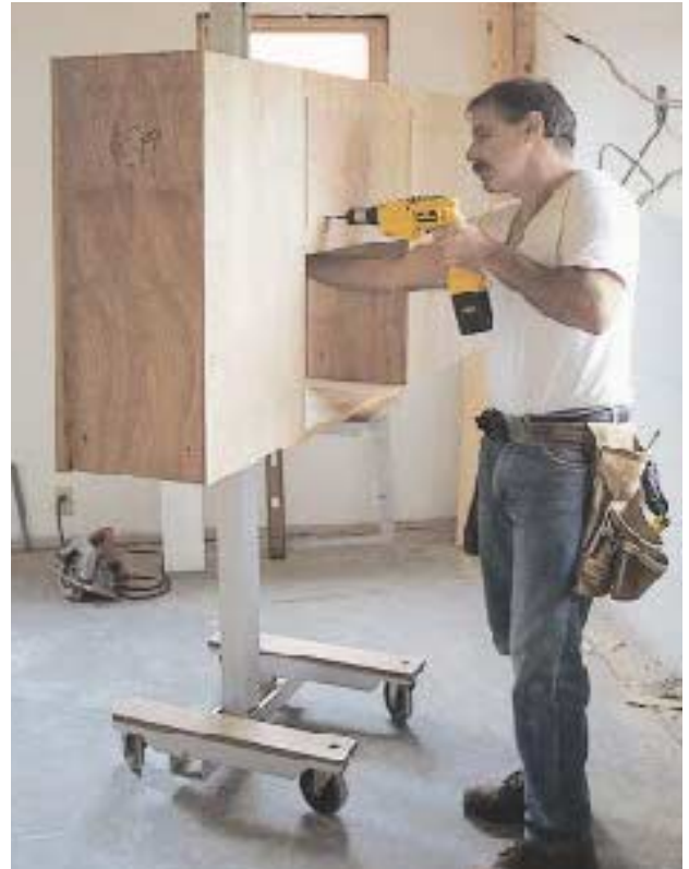
Figure 4. Marking stud locations on the backs of cabinets is easier than marking them inside (left). The author predrills holes for the mounting screws from the back (right), then finishes up with a countersink bit from the inside.
