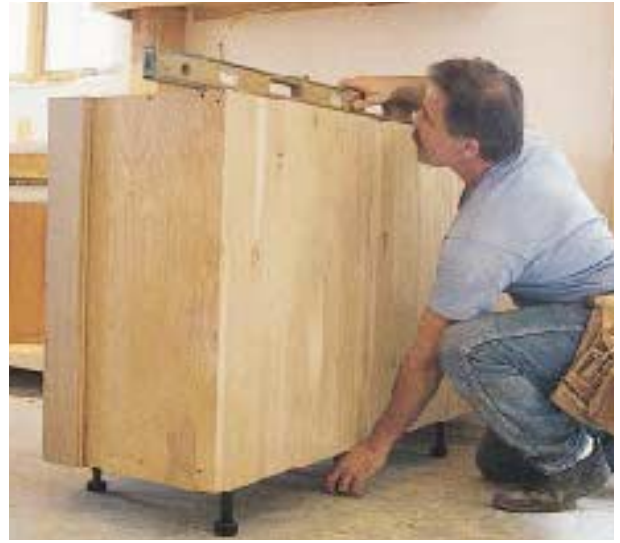
Figure 6. Plastic leg levelers (left) speed the task of leveling base cabinets (right). Finished toe kicks attach with metal clips — or can even be screwed directly into the plastic legs, according to the author.
