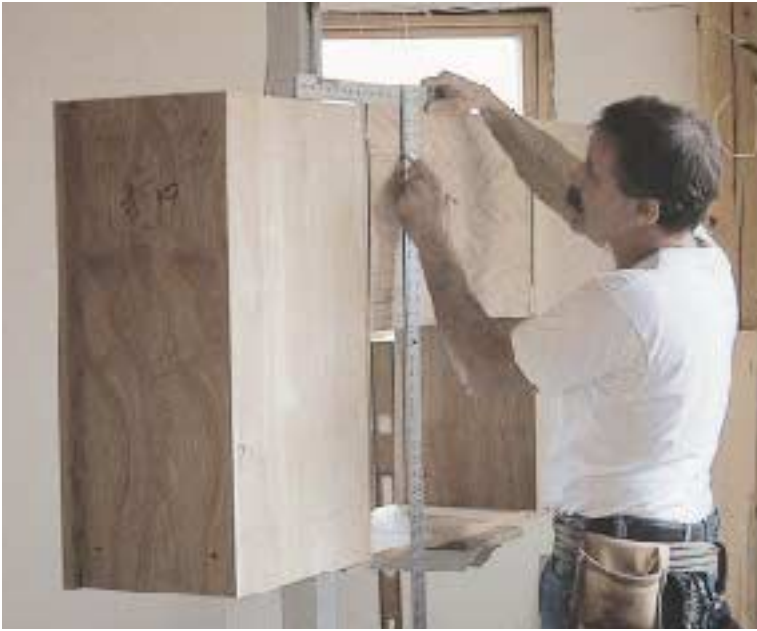
Figure 4. Marking stud locations on the backs of cabinets is easier than marking them inside (left). The author predrills holes for the mounting screws from the back (right), then finishes up with a countersink bit from the inside.
