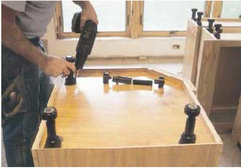
Figure 6. Plastic leg levelers (left) speed the task of leveling base cabinets (right). Finished toe kicks attach with metal clips — or can even be screwed directly into the plastic legs, according to the author.
