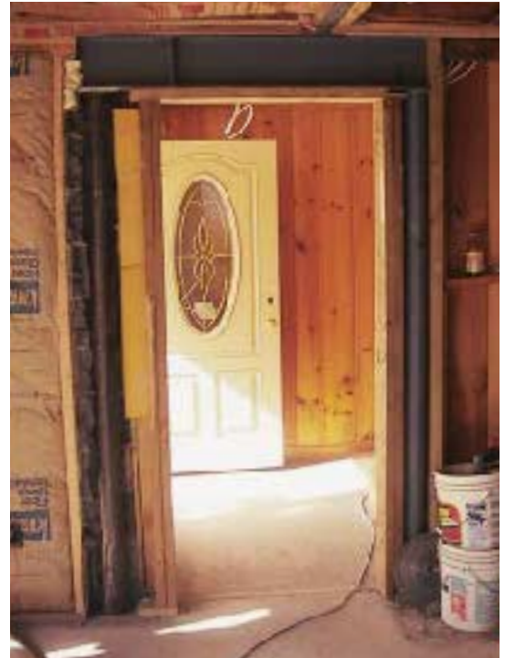
Figure 6. Metal hangers added support to the original joists as the block wall was removed (above). Installing the second column under the header allowed that section of the block wall to be removed (right).
