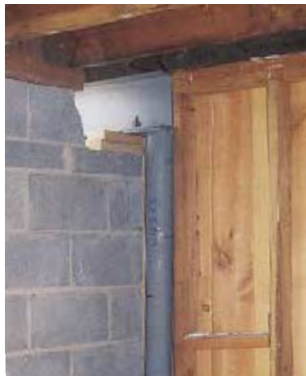
Figure 2. The steel I-beam header for the new passage door rested temporarily on the existing block wall (above) and one of two permanent steel columns (left).
