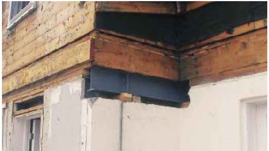
Figure 2. The steel I-beam header for the new passage door rested temporarily on the existing block wall (above) and one of two permanent steel columns (left).
