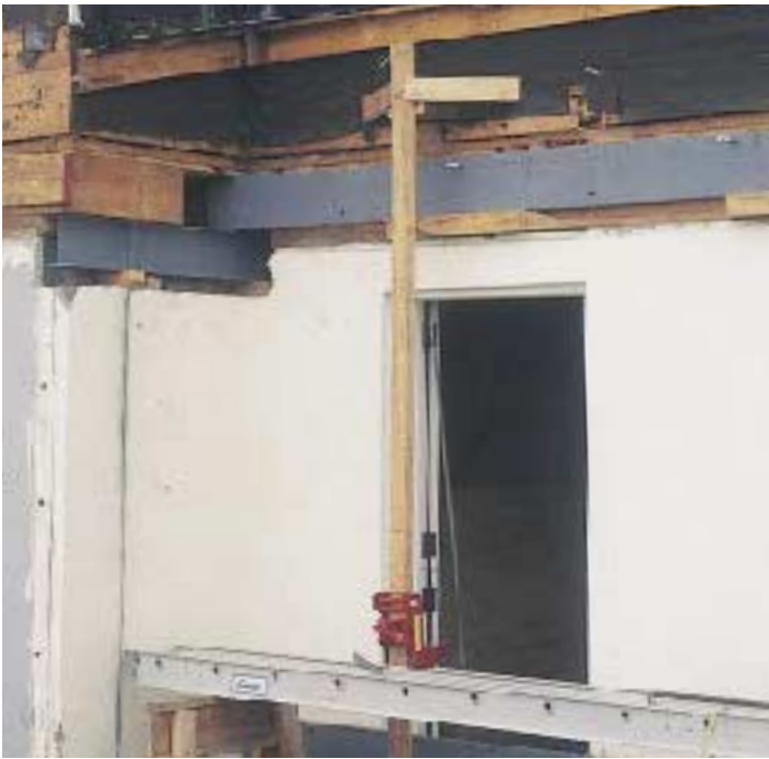
Figure 4. As the plates were lifted into place, they rested on bolts installed from the inside (left). A 2x10 completed the sandwich (right).
