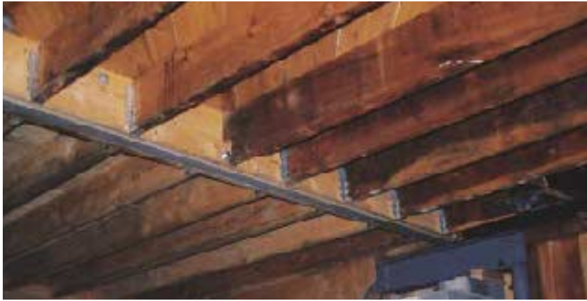
Figure 6. Metal hangers added support to the original joists as the block wall was removed (above). Installing the second column under the header allowed that section of the block wall to be removed (right).
