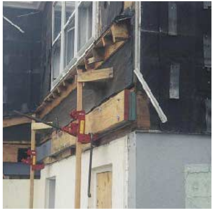
Figure 4. As the plates were lifted into place, they rested on bolts installed from the inside (left). A 2x10 completed the sandwich (right).
