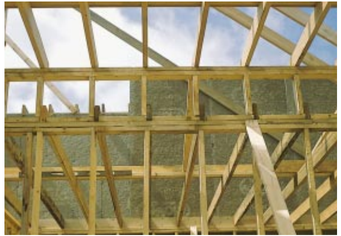
Figure 5. This short kneewall (left) is designed to add extra insulation space over the exterior wall, but it is framed only half-right. The 2x4 diagonals nailed between the top of the wall and the ceiling joists brace against outward thrust, but the wall needs to be sheathed to prevent racking. In a similar situation (right), a kneewall has been added to accommodate two different ceiling heights. The joists themselves provide resistance to any hinge action, because they are tied to an existing wall. But the wall needs drywall on both sides or plywood sheathing on the attic side, 4 feet in from each end, to prevent racking.
