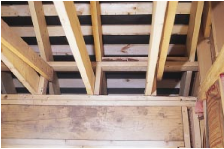
Figure 5. This short kneewall (left) is designed to add extra insulation space over the exterior wall, but it is framed only half-right. The 2x4 diagonals nailed between the top of the wall and the ceiling joists brace against outward thrust, but the wall needs to be sheathed to prevent racking. In a similar situation (right), a kneewall has been added to accommodate two different ceiling heights. The joists themselves provide resistance to any hinge action, because they are tied to an existing wall. But the wall needs drywall on both sides or plywood sheathing on the attic side, 4 feet in from each end, to prevent racking.
