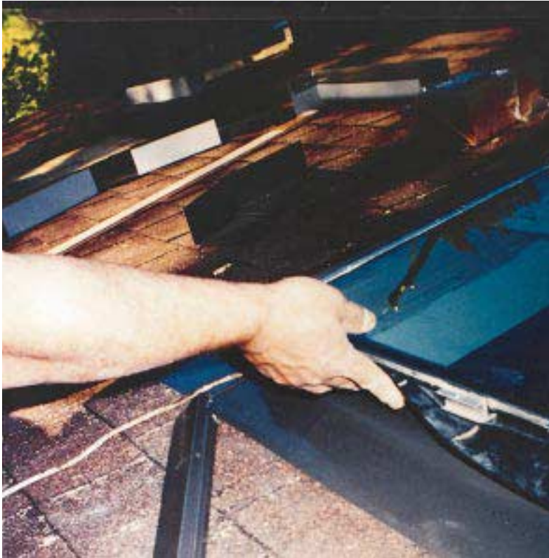
Figure 3. Prebent flashing supplied by the manufacturer tucks under a flexible rubber counterflashing gasket on this Velux unit.
