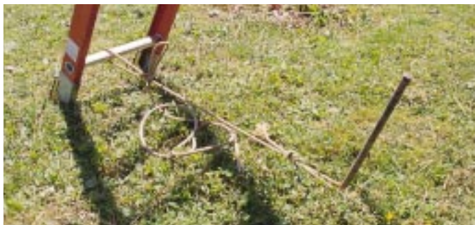
Figure 4. You can quickly secure the base of a ladder by tying off the first rung to a stake driven in the ground.
