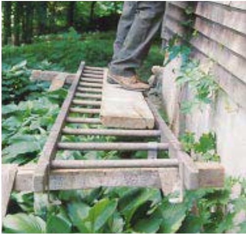
Figure 3. A shaky footing (upper left) is an accident waiting to happen. Dig out a level area and use a 2x10 pad. Driving a fastener through the ladder rail (upper right) weakens the rail and voids the manufacturer's warranty. Never use a ladder in a horizontal position (bottom left): You'll weaken the connections between the rungs and the rails, void the manufacturer's warranty, and risk an OSHA fine. Don't make creative repairs (bottom right) — you'll be assuming all the liability if the ladder fails. Instead, you should destroy the ladder.
