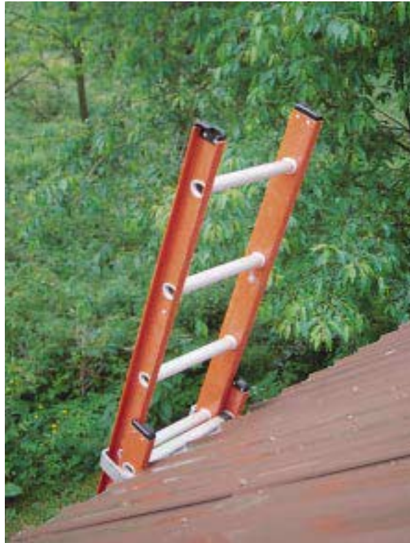
Figure 1. A ladder should extend above the eaves of a roof 3 to 3½ feet (three to four rungs).
