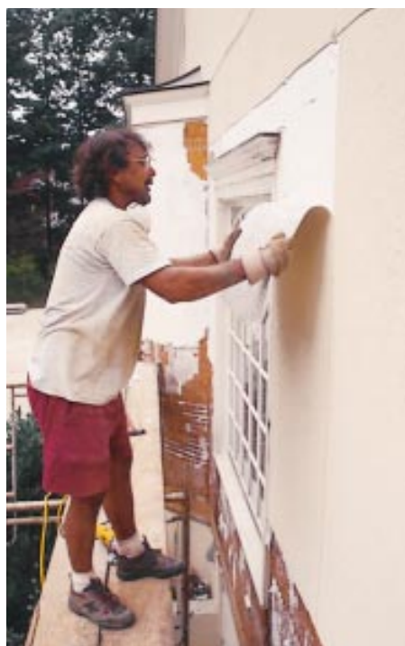
Figure 3. To remove the EIFS cladding, the author’s crew first cuts 1/4-inch-deep kerfs in the stucco skin, using a 4-inch masonry grinding wheel (left). The 3x5-foot sections or “skins” are then peeled away, exposing the underlying foam (right).
