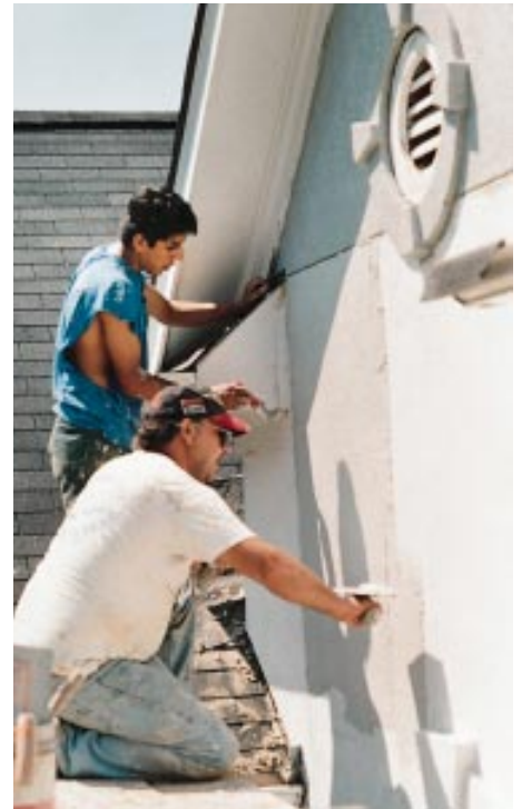
Figure 10. The base coat plaster is first used to bed all joints and to fill inside and outside corners (left). Once the bedding cures, the base coat is troweled onto an entire elevation at one time to avoid cold joints. After the base coat has cured for 24 hours, the finish coat is troweled on and textured, much like conventional stucco (right).
