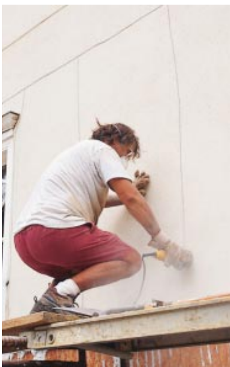
Figure 3. To remove the EIFS cladding, the author’s crew first cuts 1/4-inch-deep kerfs in the stucco skin, using a 4-inch masonry grinding wheel (left). The 3x5-foot sections or “skins” are then peeled away, exposing the underlying foam (right).
