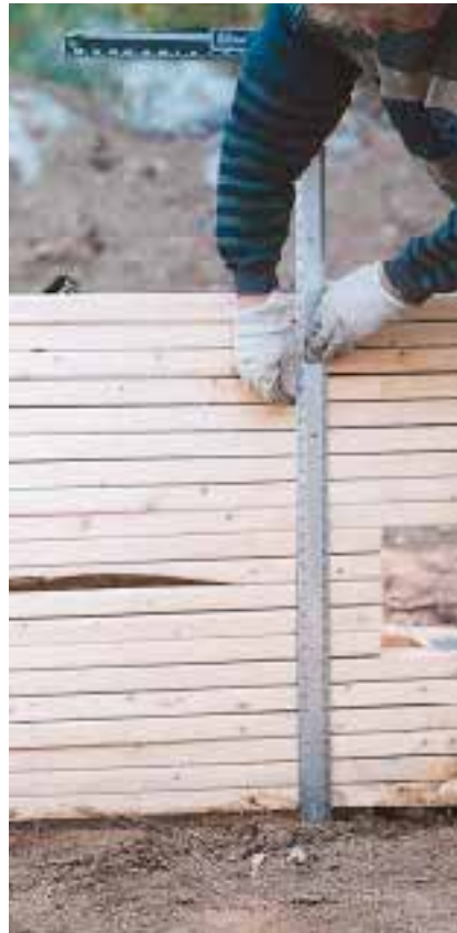
Figure 1. After the trusses are dropped on site, the crew first flushes up the stacks (top left), then marks important layout lines, including ceiling strapping (bottom left) and the exterior wall plates (near left).
