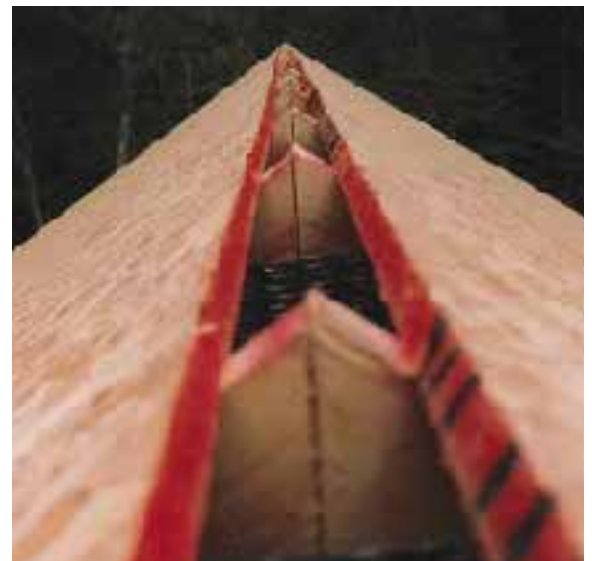
Figure 5. The sheathing is installed to premarked layout lines on the top chord. The layout is planned so that installer begins with the first full sheet at the bottom and works up (left), leaving a ventilation gap at the top (right).
