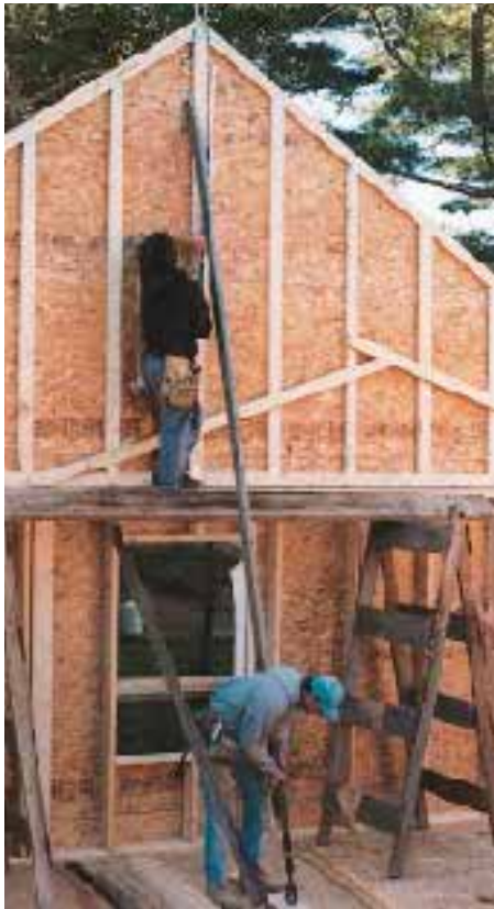
Figure 3. Gable-end trusses, which are sheathed on the ground, are set first and temporarily braced to the deck below (left). As subsequent trusses are set, steeper, more stable braces are added (right).
