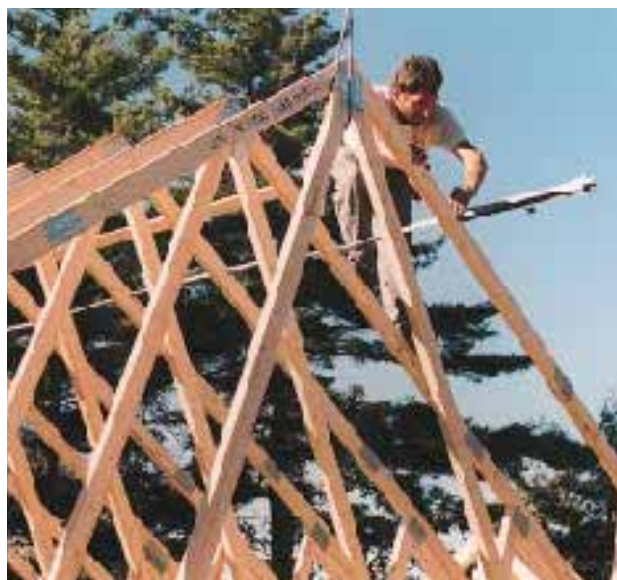
Figure 2. It takes a crew of five to set the trusses with a crane. A man on the ground attaches the crane hook and steers the truss with a tag line (top). A man at each plate positions the trusses to the layout lines, while two men above set the truss spacers (middle and bottom).
