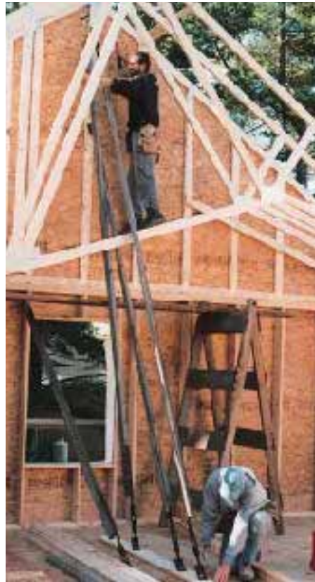
Figure 3. Gable-end trusses, which are sheathed on the ground, are set first and temporarily braced to the deck below (left). As subsequent trusses are set, steeper, more stable braces are added (right).
