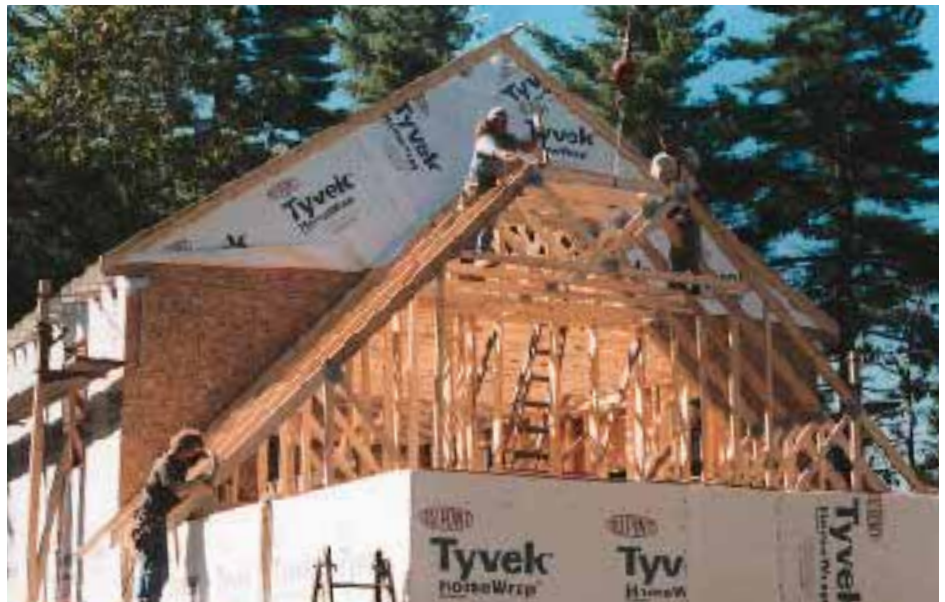
Figure 2. It takes a crew of five to set the trusses with a crane. A man on the ground attaches the crane hook and steers the truss with a tag line (top). A man at each plate positions the trusses to the layout lines, while two men above set the truss spacers (middle and bottom).
