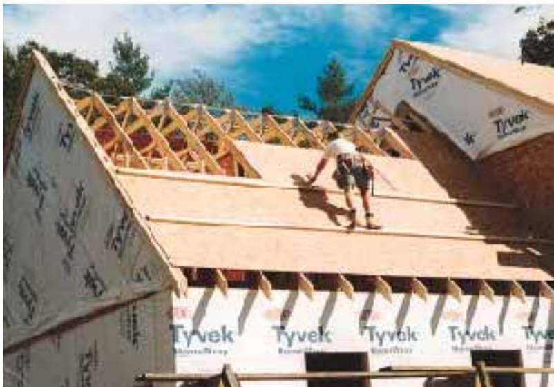
Figure 5. The sheathing is installed to premarked layout lines on the top chord. The layout is planned so that installer begins with the first full sheet at the bottom and works up (left), leaving a ventilation gap at the top (right).
