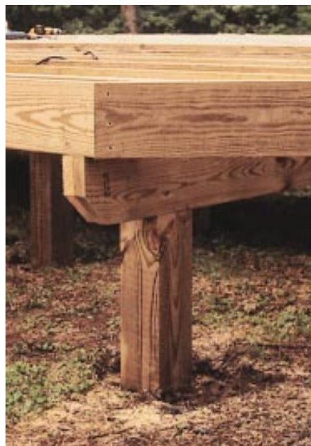
Figure 2. The author notches carrier beams into the 6x6 support posts (left). The ends of the beams are clipped for a nicer appearance (above).
