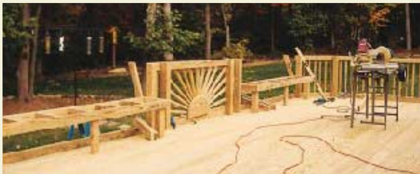
The sunrise pattern and built-in benches are two of the details the author uses to set his decks apart.
