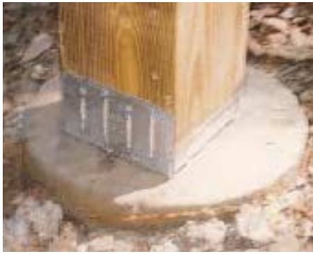
Figure 1. Galvanized post anchors make for a secure attachment to concrete pier footings and help prevent decay at the bottom of the post.
