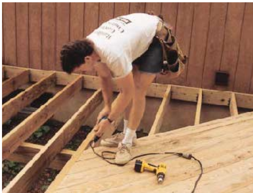
Figure 4. The author uses a raised joist with 2x6 cleats on both sides to catch the ends of angled or straight-run decking boards. This detail breaks up the decking into smaller areas and avoids the use of splices in the deck boards.
