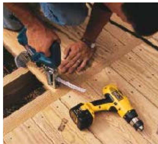
Figure 4. The author uses a raised joist with 2x6 cleats on both sides to catch the ends of angled or straight-run decking boards. This detail breaks up the decking into smaller areas and avoids the use of splices in the deck boards.
