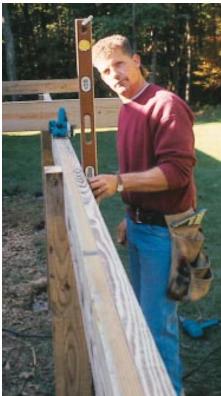
Figure 2. The author notches carrier beams into the 6x6 support posts (left). The ends of the beams are clipped for a nicer appearance (above).
