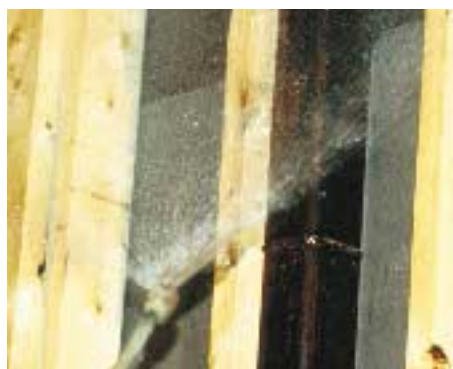
Figure 1. For an effective treatment against termites and carpenter ants, PCOs spray all framing and sheathing surfaces with a borate solution at the "dried-in" stage of construction. The low-pressure sprayer uses a wide nozzle to deliver a fan-shaped spray (above).
