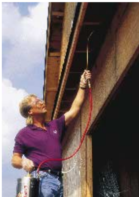
Figure 1. For an effective treatment against termites and carpenter ants, PCOs spray all framing and sheathing surfaces with a borate solution at the "dried-in" stage of construction. The low-pressure sprayer uses a wide nozzle to deliver a fan-shaped spray (above).
