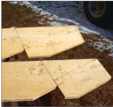
Figure 4. When laying out seat cuts, it is critical to maintain the same height above the plate on both hip and common rafters.
