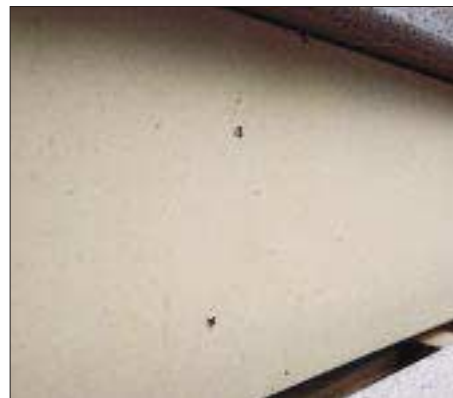
Figure 4. When a finish nail is set in PrimeTrim, it leaves a pucker that must be sanded and primed to leave a smooth finished surface.
