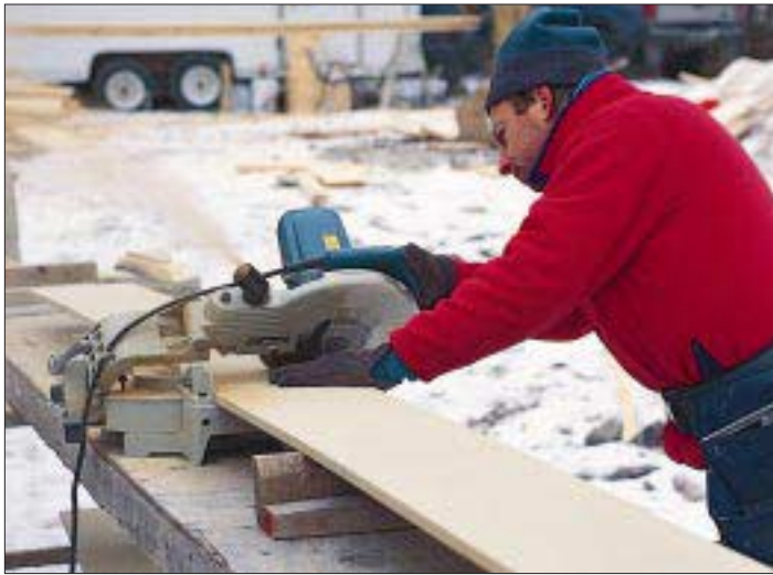
Figure 3. Although it can be cut with ordinary tools, PrimeTrim is very hard and dulls even carbide-tipped blades much more quickly than solid wood.
