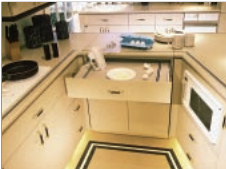
Figure 3. Adding lights to this toe space and turning the drawer into a slide-out counter made life easier for a wheelchair user. But universal design ideas like these also go a long way toward dressing up any kitchen.
