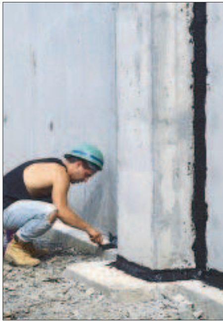
Figure 2. Sheet membranes give consistent coverage to both walls and footings (far left). Some manufacturers require you to smooth all inside corners with a troweled mastic before installing the membrane (middle). Membrane edges must also be sealed with mastic (above).
