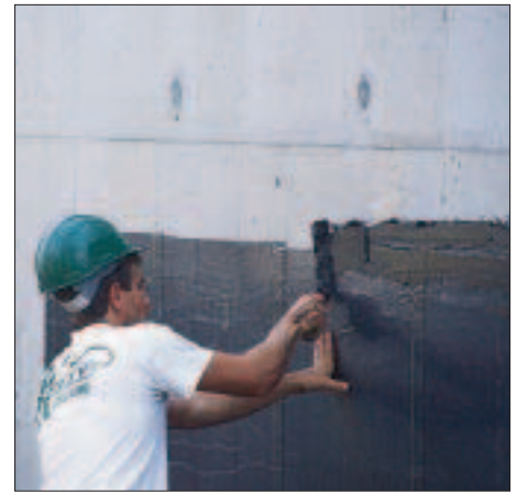
Figure 2. Sheet membranes give consistent coverage to both walls and footings (far left). Some manufacturers require you to smooth all inside corners with a troweled mastic before installing the membrane (middle). Membrane edges must also be sealed with mastic (above).
