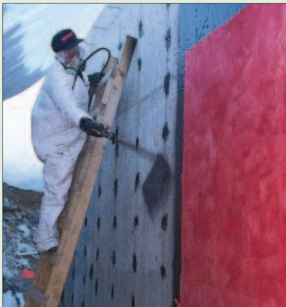
This Tuff-N-Dri installer is protected from head to toe — the high-pressure spray gun can inject chemicals directly through the skin into the blood.
