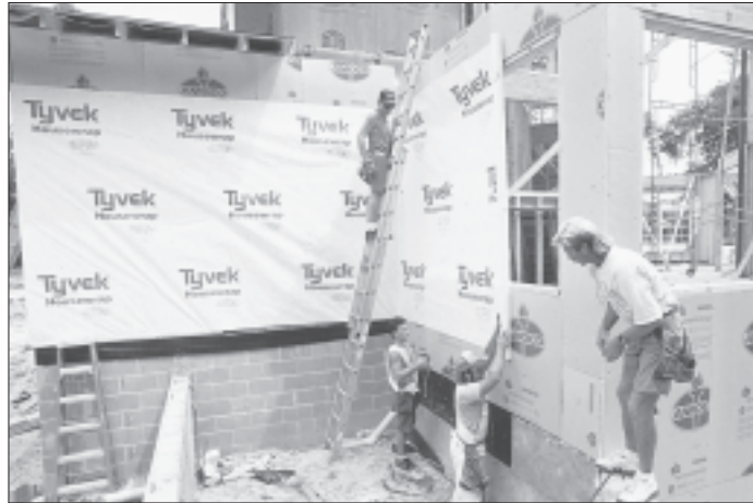
Builders have questioned the practice of installing housewrap over foam sheathing, but DuPont says laboratory data show that it helps (see chart, below).
