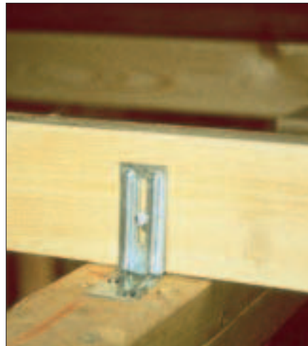
Figure 7. Most roof trusses are designed to bear only at the exterior walls. Avoid nailing roof trusses to interior partitions (far left); otherwise, as the bottom chord rises with changes in moisture content, it will move the wall with it and open up cracks in the ceiling drywall. Instead, use truss clips (left), which allow the truss to move independently of the partition wall.
